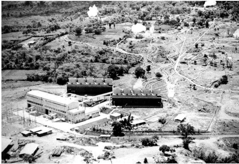
Figure 8.2 Ahuachapan geothermal facility after commissioning around 1977 (DiPippo, 1978).
