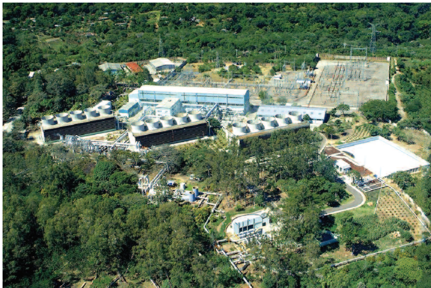
Figure 8.3 Ahuachapan geothermal facility after revegetation, circa 2005 (LaGeo, 2005).
