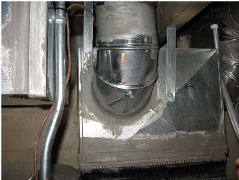
Figure 14. Typical ductwork sealing at takeoff from trunk; elbow to the site is sealed
