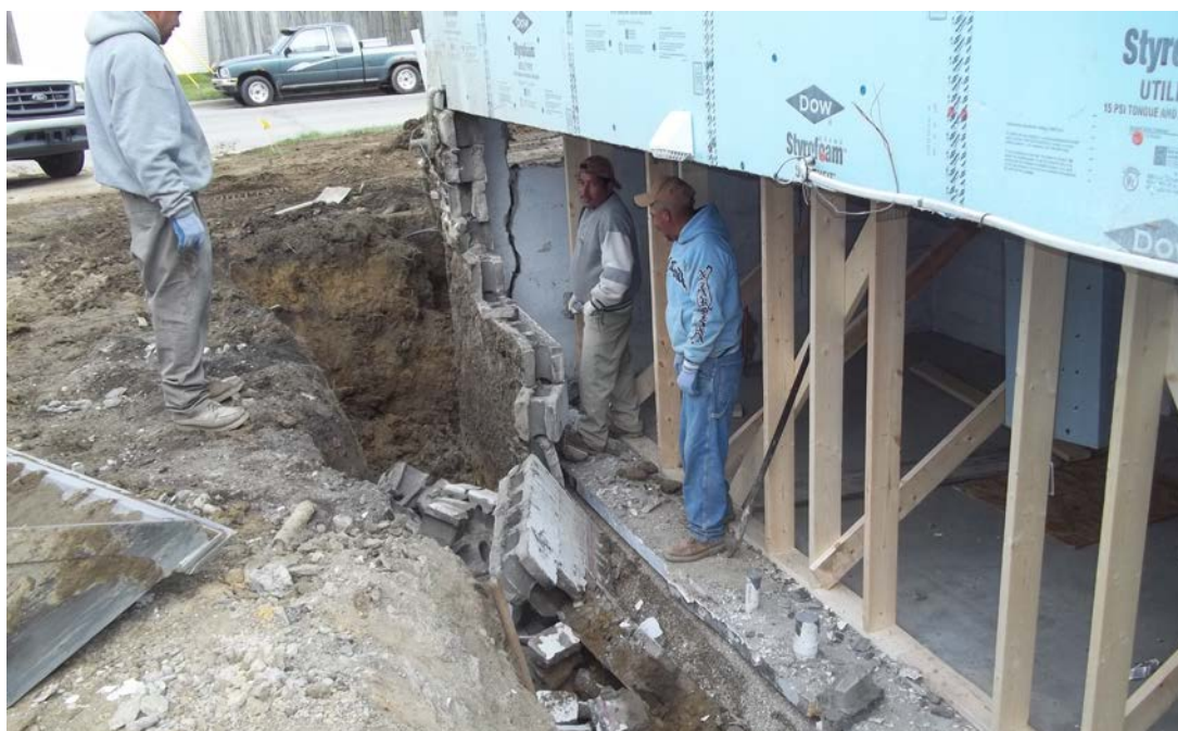
Figure 5: Repair work on Cedar 2 foundation
