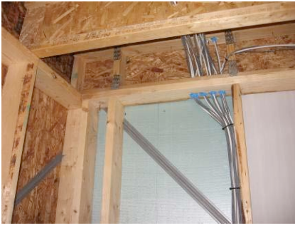
2011-10-06 – Mechanical and electrical work continues
