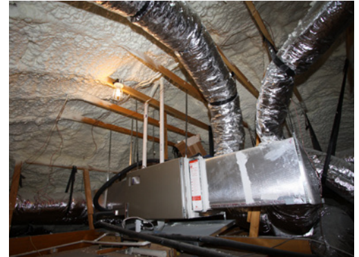
(Top) Spray foam insulation. Spray foam was used to simultaneously air seal and insulate this ventilated attic. Baffles installed in each rafter bay keep the insulation from blocking the soffit vents (Photo Source: WSU Energy Office).
