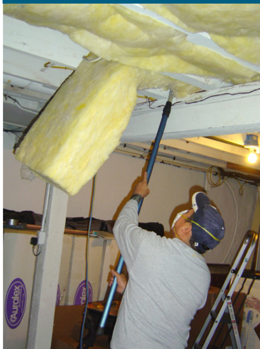
Basement ceiling insulation. Unfaced fiberglass batts are installed in the ceiling of this basement in Portland, Oregon (Photo Source: PNNL).
