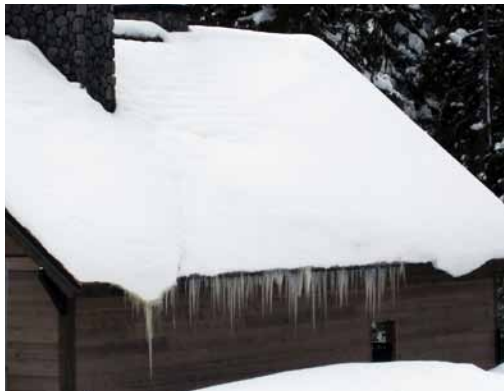
Icicles indicate ice dams are forming (Photo Source: PNNL).
