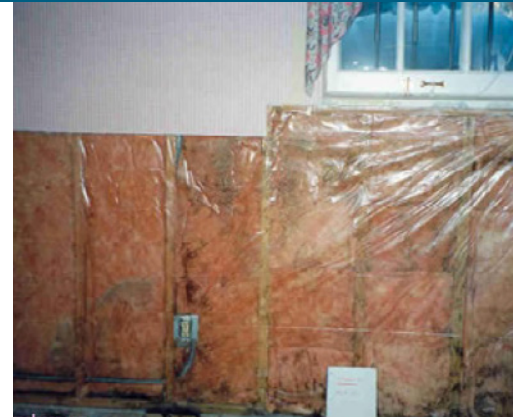
Vapor retarders and mold. Vapor barriers like this polyethylene sheet can trap moisture in walls. The damp fiber insulation in this wall developed mold and odors (Source: BSC).
