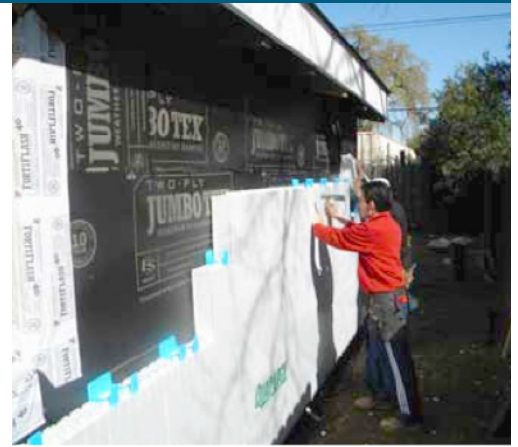
Exterior foam block insulation.
