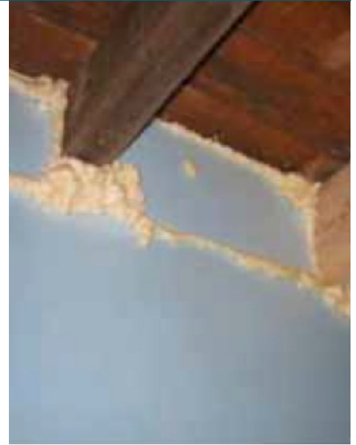
Interior rigid foam. To create an air barrier, seams of the rigid foam insulation were carefully sealed with spray foam (Photo Source: PNNL).
