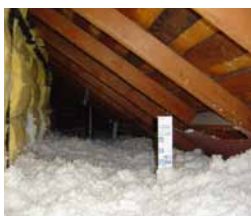
This attic kneewall has been thoroughly insulated.
