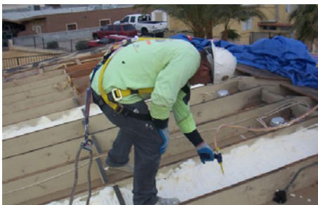
Closed-cell spray foam fills the rafter bays of the vented cathedral ceiling.
