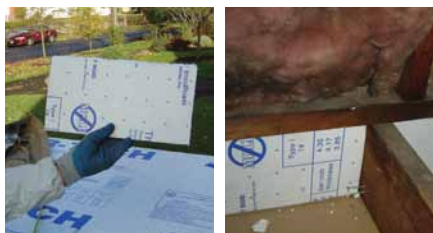
Figure 4. Air seal floor joist cavities under kneewalls by filling the cavities with rigid foam insulation, OSB, or another rigid material that is cut to fit and sealed at the edges with caulk (as shown here and below). Another option is to block the joist cavity with fiberglass batts that are rolled and stuffed in plastic bags or covered with spray foam.
