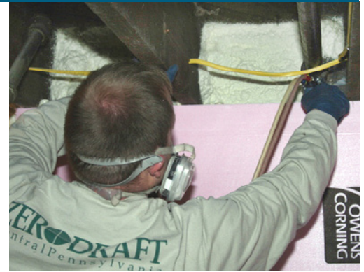
Basement wall insulation. In this Pennsylvania basement, rigid XPS foam insulation is attached directly to the concrete basement walls with spray foam. Rim joists are insulated with spray foam. Frame walls will be built to finish the basement (Photo Source: Asdal Construction).
