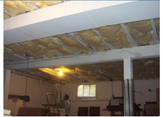
Basement ceiling insulation. When this home was remodeled for energy efficiency, the basement ceiling was extensively air sealed and then insulated with unfaced batts (Photo Source: PNNL).
