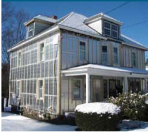
Exterior rigid insulation. A complete renovation of this Massachusetts home included insulating the walls with exterior rigid insulation and interior cellulose (Photo Source: BSC).
