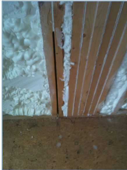
Figure 3. Over-designed framing at panel juncture
