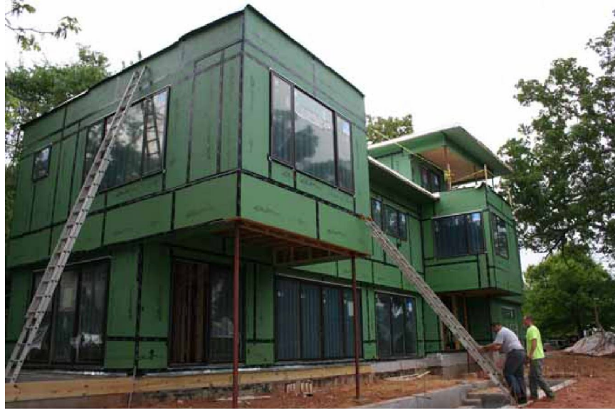
Figure 5. Taped exterior sheathing panels
