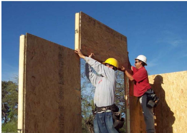
Figure 3. SIP wall installation
