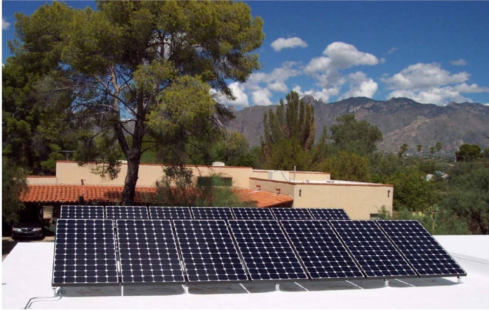
Figure 7. The 3kW photovoltaic system
