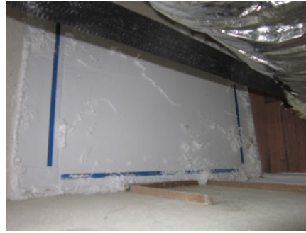
Figure 12. After: Opening in wall above dropped ceiling patched and sealed
