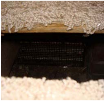
Figure 5. Before: Disconnected duct boot behind floor register
