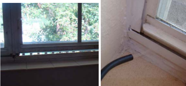
Figure 15. Before: Old windows not closing tightly
