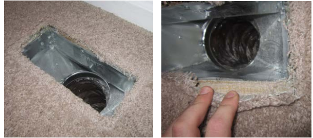
Figure 6. After: Boots sealed to subfloor
