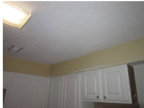
Figure 8. After: New gypsum board ceiling in kitchen isolates wall penetrations from living space
