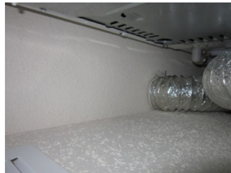
Figure 10. After: Sealed wall above dropped ceiling
