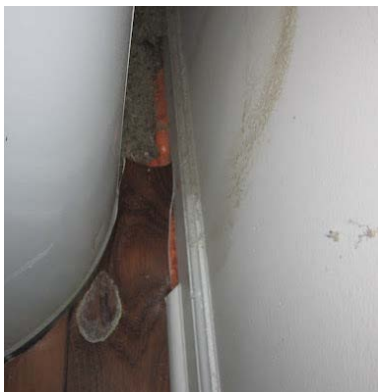
Figure 25. After: Crack under wall in mechanical space sealed to floor with foam
