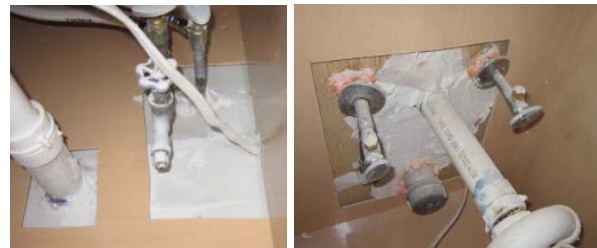
Figure 18. After: Plumbing penetrations sealed around pipes and behind escutcheons with foam and caulk
