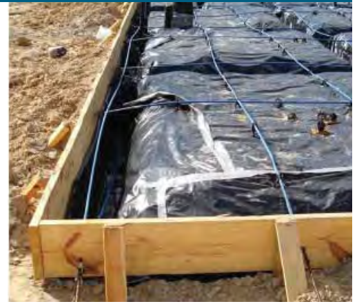
David Weekley Homes uses a slab foundation including a 4-in.-thick post-tensioned monolithic slab with turned-down edges poured over 6-mil polyethylene, which serves as a capillary break. Slab edge insulation is not used due to termite risk.
