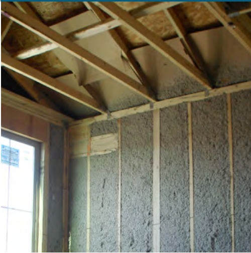
Baffles allow ventilation under roof decking while keeping wind from blowing insulation back from the edges of an attic.
