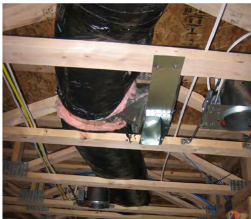
(Top and Bottom) These Building America builders run ducts through open-web floor trusses to keep the ducts in conditioned space. Open-web trusses allow subcontractors the flexibility to run plumbing, electrical, and ductwork easily between floors, with little to no “trade damage” or “trade fighting.” Air handlers are located in conditioned space in the home or in an air-sealed closet in the garage.
