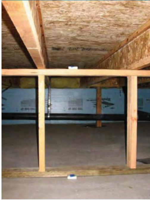
Unvented, insulated crawlspaces are recommended in the eastern and midwestern United States, where high humidity levels can cause moisture problems in vented crawlspaces.
