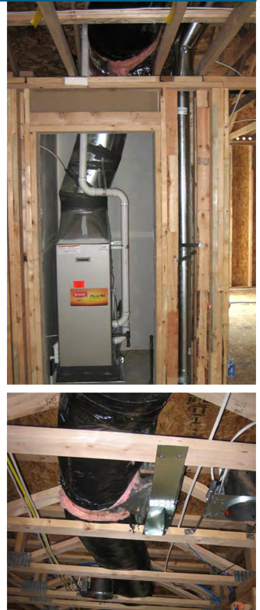
(Top and Bottom) These Building America builders run ducts through open-web floor trusses to keep the ducts in conditioned space. Open-web trusses allow subcontractors the flexibility to run plumbing, electrical, and ductwork easily between floors, with little to no “trade damage” or “trade fighting.” Air handlers are located in conditioned space in the home or in an air-sealed closet in the garage.
