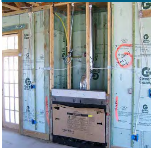
Rigid foam insulates the interior of masonry walls behind the fireplace in this Building America home by Castle and Cooke in Winter Garden, Florida.
