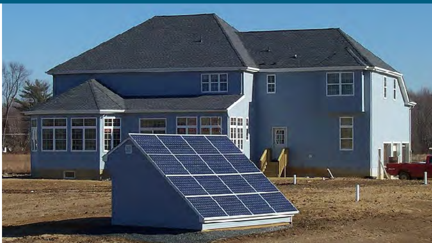
Tindall Homes installed their optional grid-tied solar photovoltaic systems on backyard garden sheds, situated for maximum solar gain. Wiring for the systems runs underground from the shed to the home's basement.
