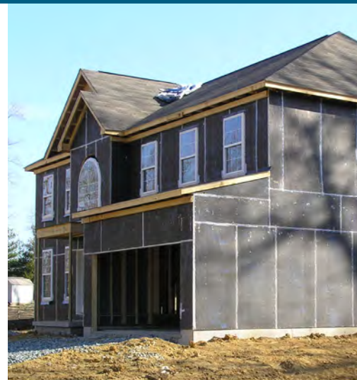
Bob Ward Companies used an exterior wall sheathing consisting of a 1/8-inch layer of laminated fiberboard covered with 1-inch of extruded polystyrene foam board. This layer goes on the exterior side of the studs under the stone or wood siding. Joints are taped so the foam board serves as an air barrier as well, eliminating the need for housewrap. This exterior insulation layer moves the dew-point surface to the outside of the framing member, reducing the potential for condensation and moisture damage within the wall cavity. (Photo source: Bob Ward Companies)
