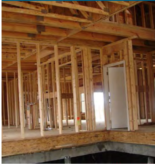
Insight Homes used advanced framing and located high-efficiency furnaces and ducts in a sealed, insulated crawlspace in its homes in Sussex County, Delaware. (Photo Source: Insight Homes)
