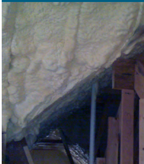
Unvented attics insulated with R-30 low-density spray foam provide a semi-conditioned space for the high-efficiency heat pump and ducts.
