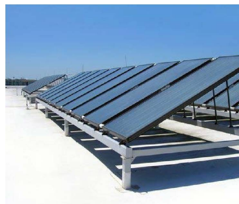
Figure 5. Commercial SWH system – IKEA Orlando
