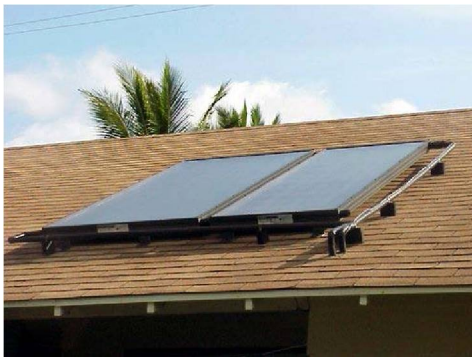
Figure A–1. Glazed flat-plate collector. Photo by Christopher Drake, NREL/PIX 09188
