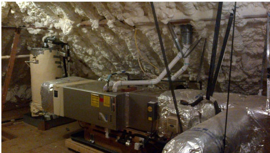
Figure 1. Non-vented attic houses equipment and ducting
