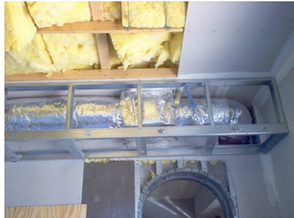
Figure 2. Duct chases in conditioned space
