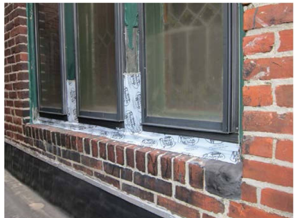
Figure 39. Rowlock window sill examples
