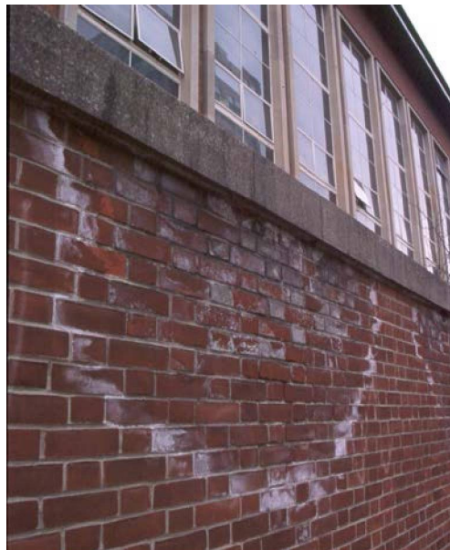
Figure 35. Failed mortar joint at sill from concentrated runoff, resulting in brick failure
