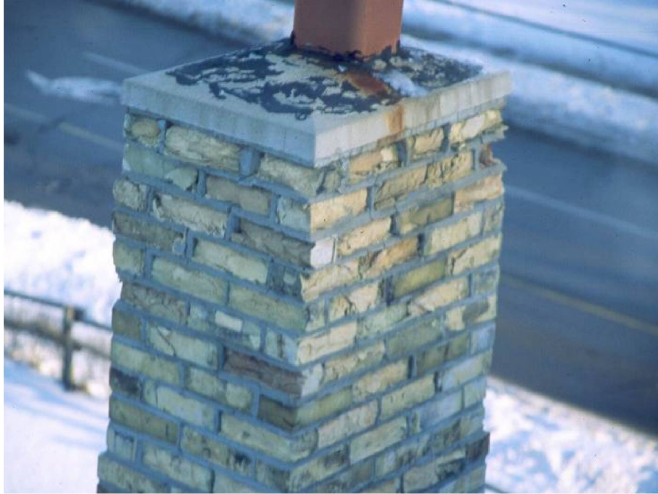
Figure 59. Severe FT damage at existing chimney; lack of projecting cap with drip edge
