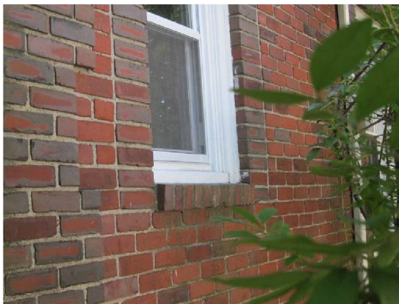
Figure 39. Rowlock window sill examples
