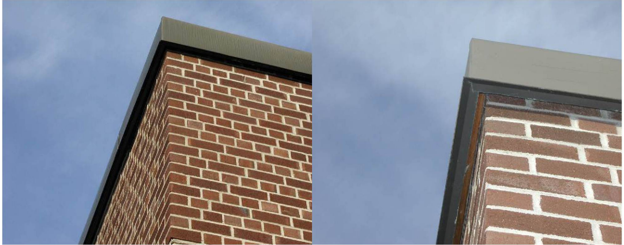
Figure 62. Improved drip edge overhang at coping
