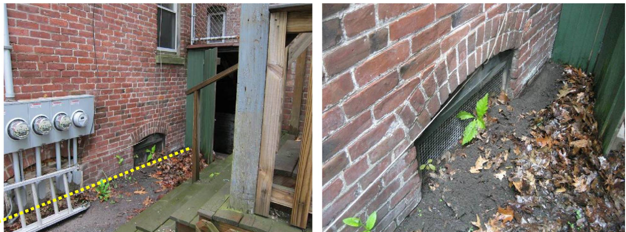
Figure 70. Left: Rear wall near subfluorescence damage visible in basement; Right: Buried window
