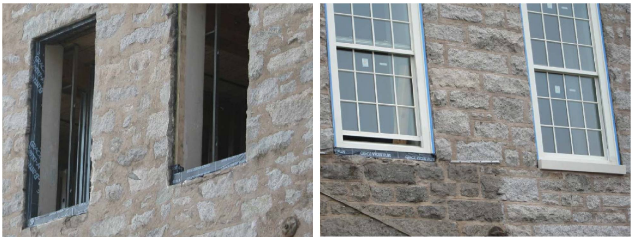
Figure 45. Left: Membrane flashing wrapping window opening; Right: Exterior view of window assembly and completed unit
