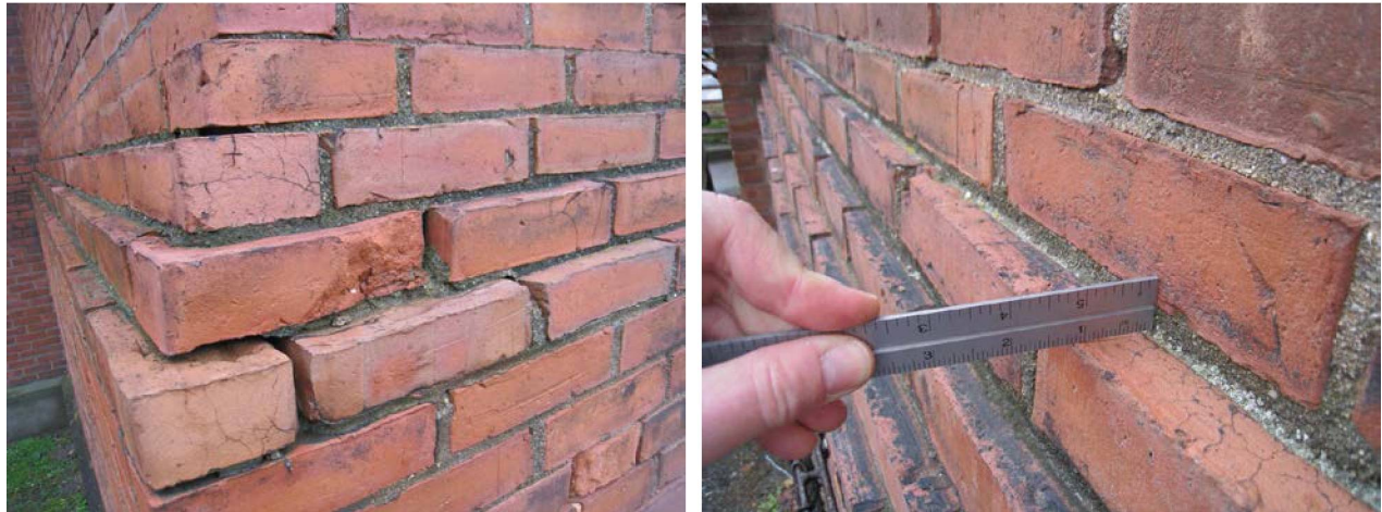
Figure 50. Steps in brickwork, and related cracking/FT damage
