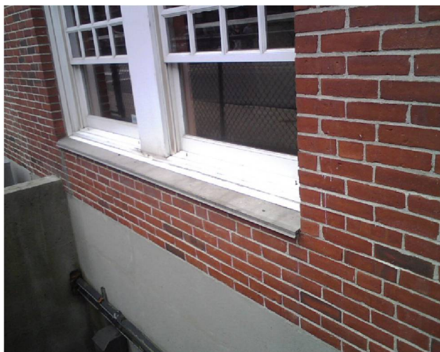
Figure 42. Example of overlaid sill detail (formed metal)
