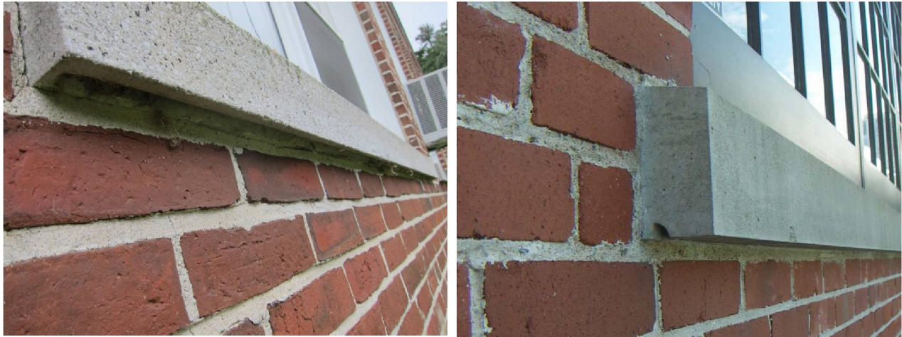
Figure 36. Precast window sill drip edge details
