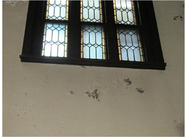
Figure 40. Left: Rowlock window sill with no projection; Right: Water deposition on wall below
