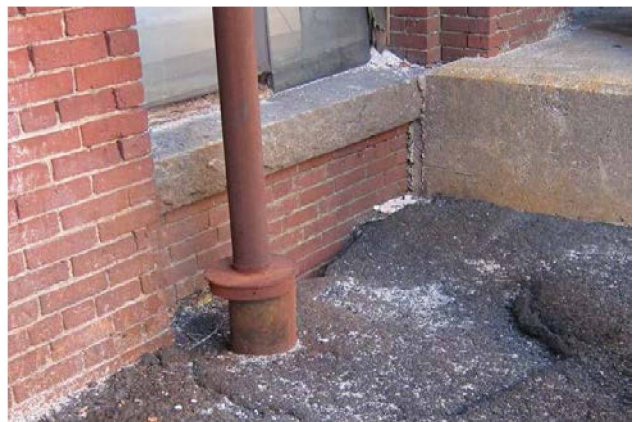
Figure 72. Exterior parking lot grade relative to interior conditions
