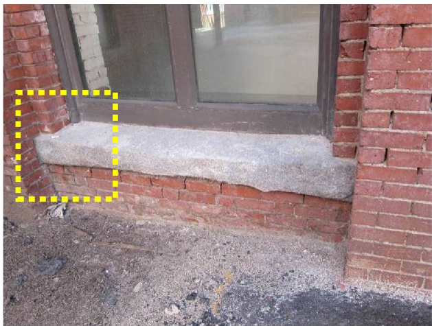
Figure 33. Solid granite sloped sill, potential for water introduction into wall
