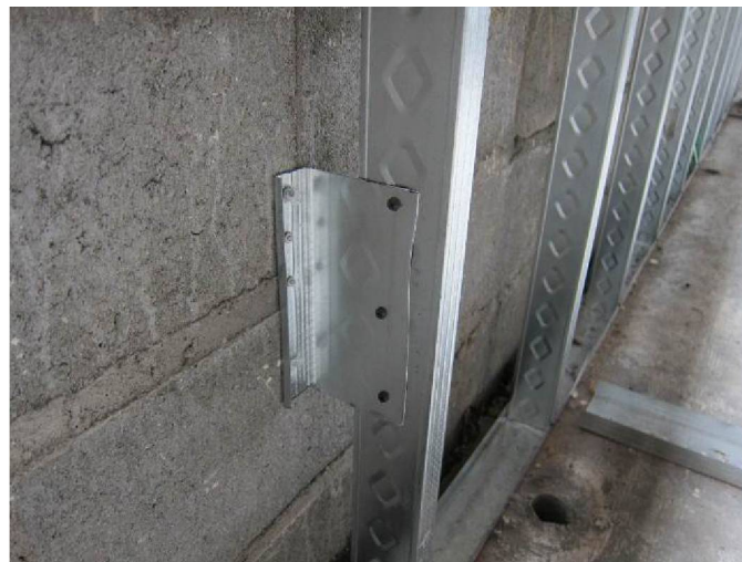
Figure 27. Clip tying framing to concrete masonry unit backup wall, steel clip shown; not recommended
