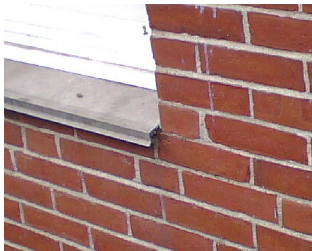
Figure 42. Example of overlaid sill detail (formed metal)
