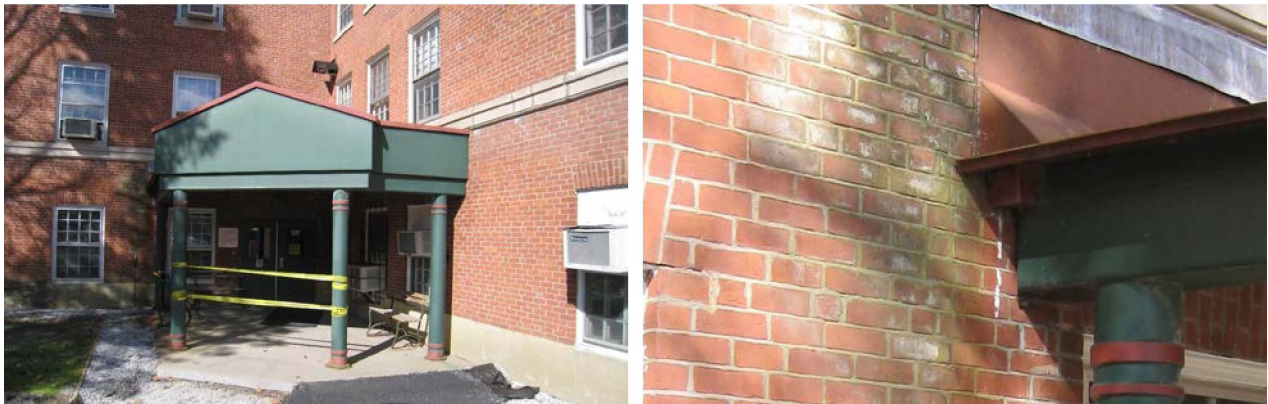
Figure 53. Left: Retrofit roof over entrance; Right: Water runoff concentration at roof-wall interface
