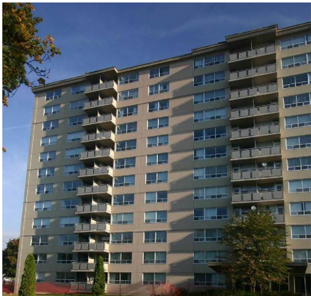
Figure 4. Exterior insulation retrofit overclad
