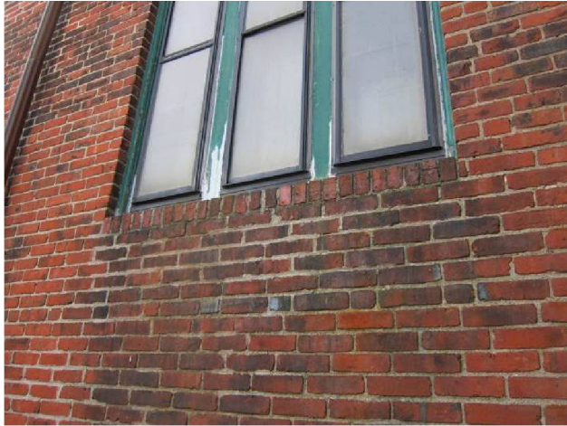
Figure 40. Left: Rowlock window sill with no projection; Right: Water deposition on wall below
