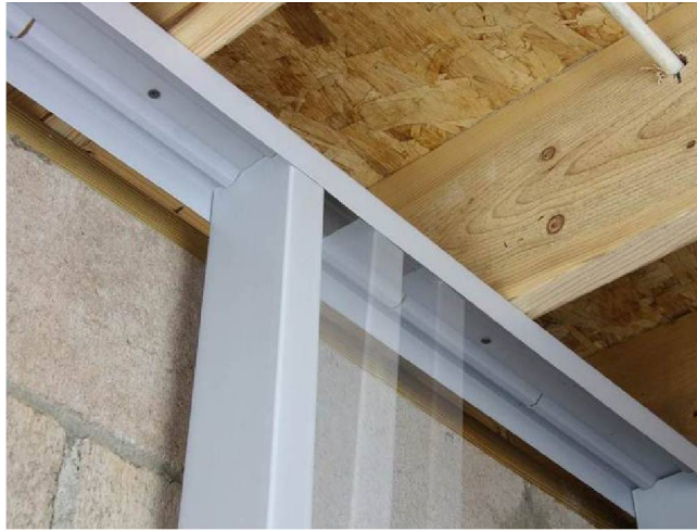
Figure 28. Polymer framing as alternate material with better thermal resistance
