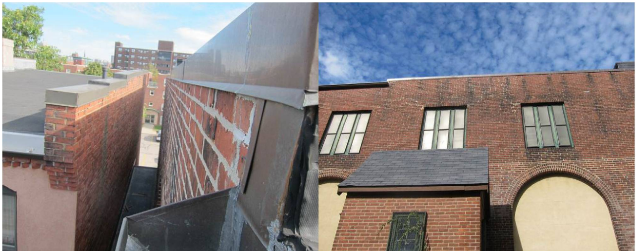
Figure 60. Coping detail and runoff staining at joints of previous coping design
