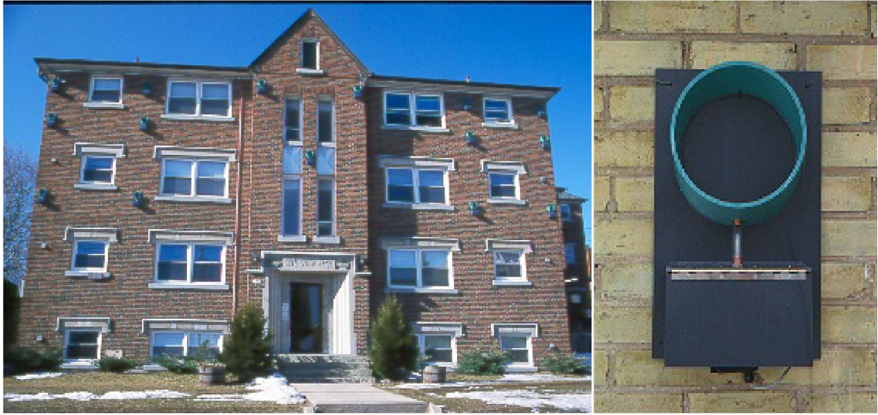
Figure 91. Instrumented occupied building (Waterloo, Ontario) with driving rain gauges
