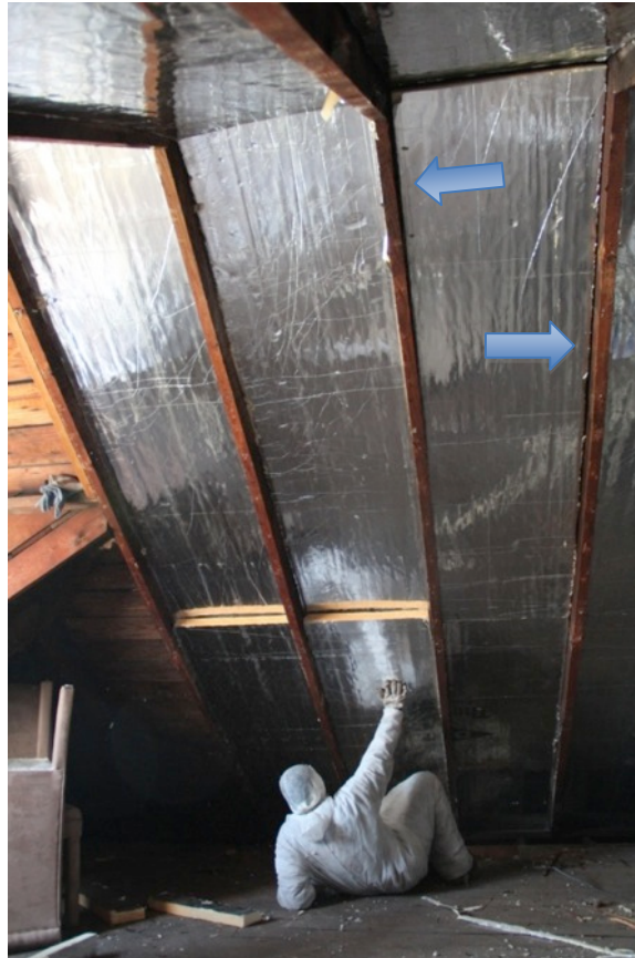
Figure 23. Foil-faced polyisocyanurate insulation fit into rafter framing cavities (Photo credit: S. Marchese, printed with permission)
