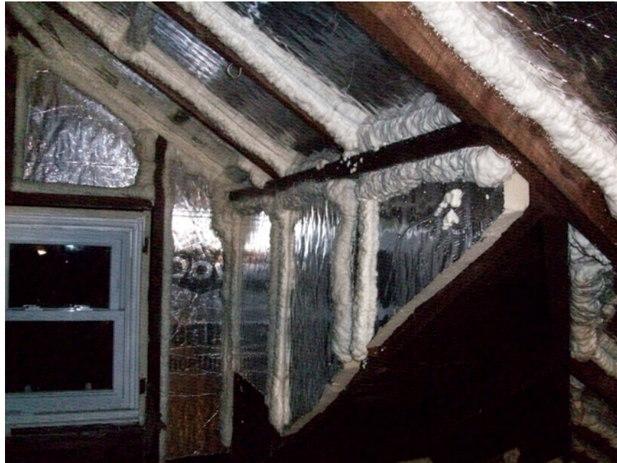
Figure 24. Foam sealant applied to seal foil-faced polyisocyanurate to surrounding framing. In this image the application of rigid insulation and foam sealant is not complete. (Photo credit: E. Haber, printed with permission)
