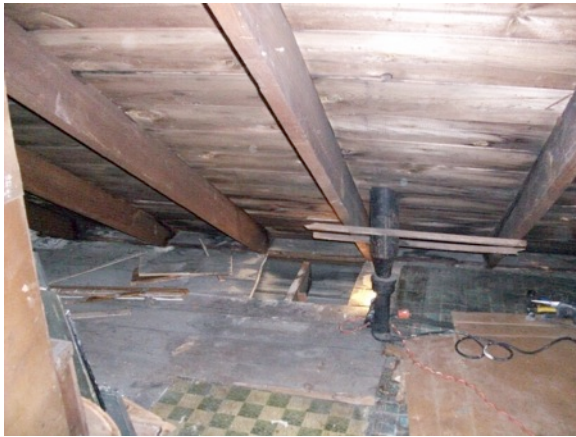
Figure 3. Left: Attic floorboards removed to investigate conditions at top of wall during assessment of prototype house; Right: Attic floorboards removed to allow access to top of wall
