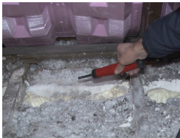
Figure 12. CEDA Weatherization assessing effectiveness of air seal at furring cavity between brick masonry and interior finish (Photo credit: S. Marchese, printed with permission)
