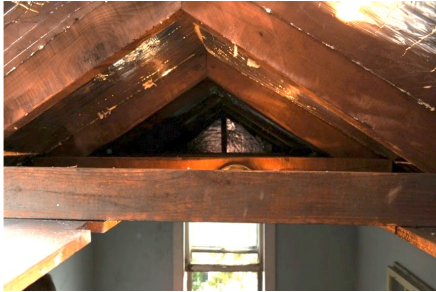
Figure 22. Foil-faced polyisocyanurate insulation installed above ceiling of finished room in attic (Photo credit: E. Haber, printed with permission)
