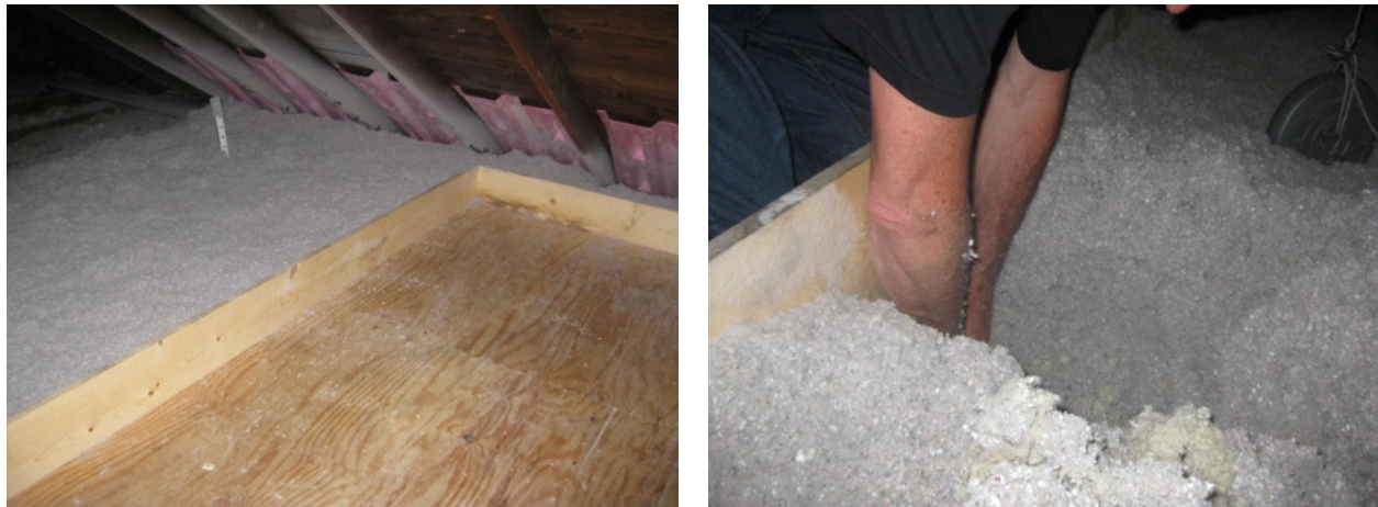
Figure 16. Left: Attic storage platform with insulation dams at the perimeter; Right: A CEDA Weatherization team member checks the depth of insulation beneath platform
