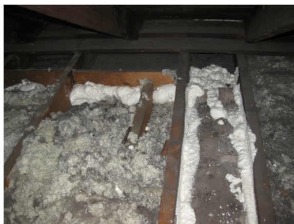
Figure 9. Left: Creating access to dropped soffit area and plumbing wall; Right: Attic floorboard repurposed in sealing plumbing chase (Photo credit: S. Marchese, printed with permission)
