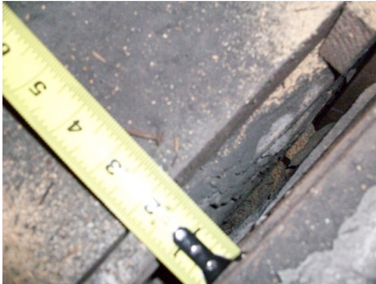
Figure 2. Furring cavity between brick masonry and interior finish as seen from the attic
