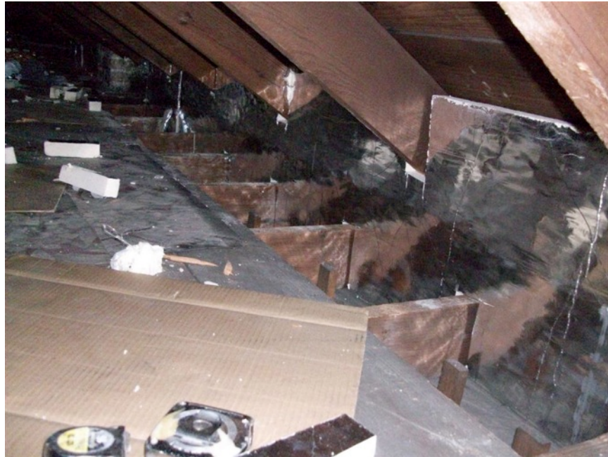
Figure 4. Foil-faced polyisocyanurate board insulation installed to transition thermal control from top of masonry wall to roof. The rigid insulation board rests on top of a wood plate at the top of the brick wall. Note that furring cavity gap (at junction of wall plaster and ceiling plaster) is to interior side of the rigid board insulation as indicated by wood furring extending above the top of the brick wall.
