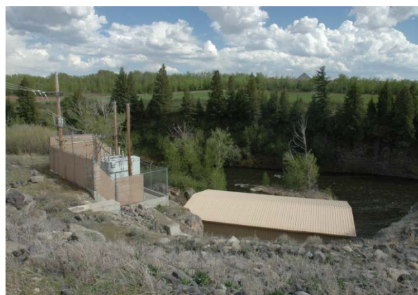
Figure 8-8. Small hydroelectric plant
