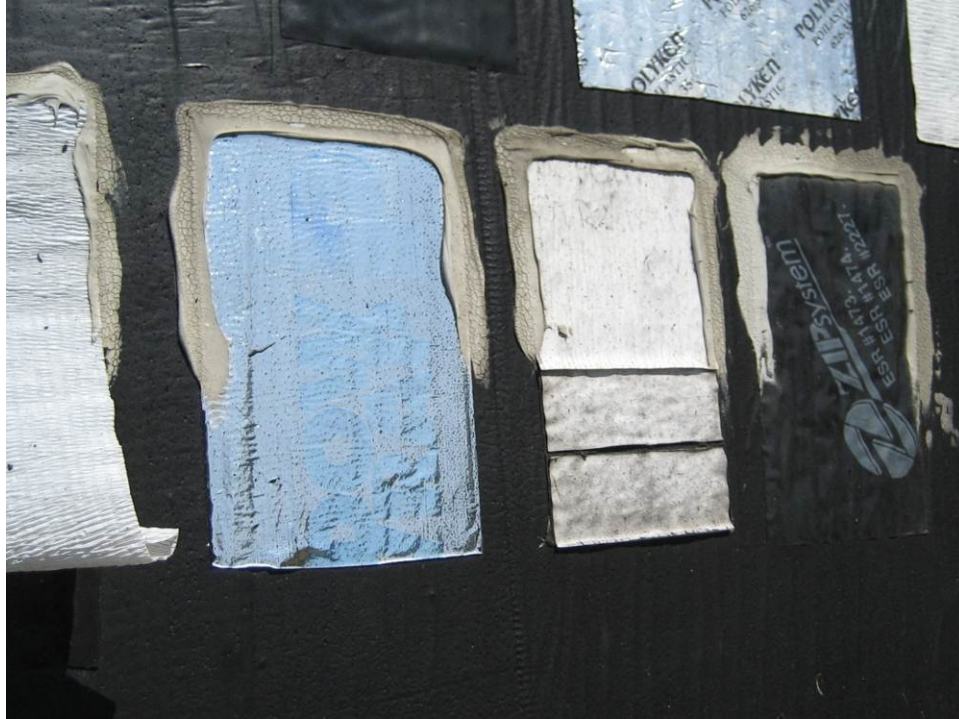
Figure 22. Peel and stick membranes with termination mastic
