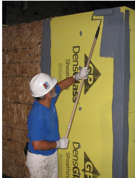
Figure 14. Roller applied liquid applied barrier
