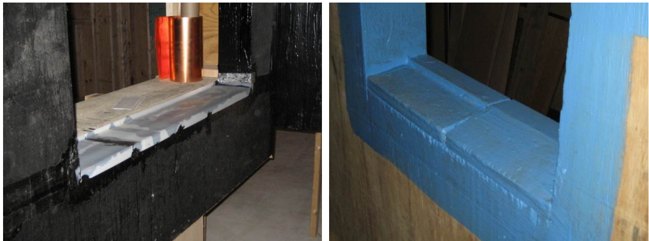
Figure 20. Window sill flashing mockups
