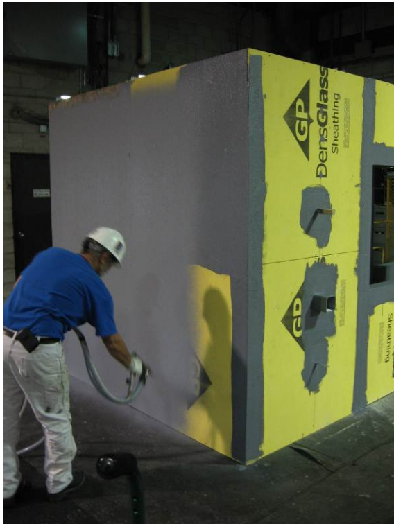
Figure 13. Spray applied liquid applied barrier
