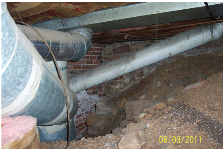
R-19 insulation is installed between the floor joists in the ceiling of this crawlspace but gets no credit on the SmartRegs checklist because heating ducts are present.
