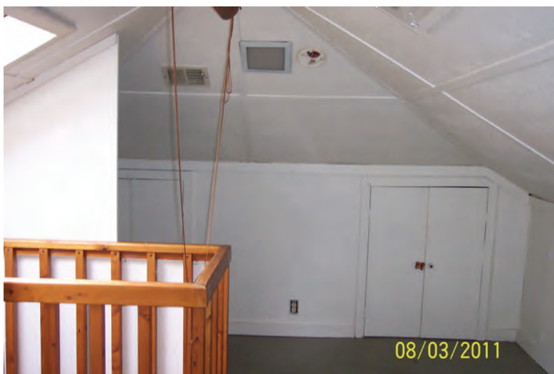
Attic is only insulated to R-11. Kneewall access hatches are extremely leaky.
