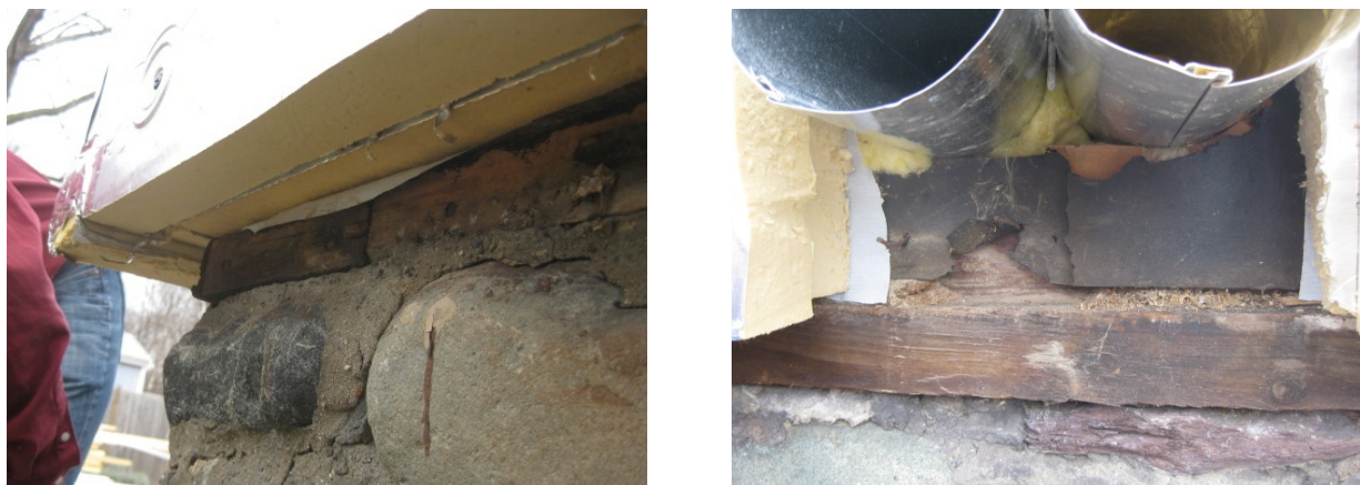
Figure 38. Left: Exterior insulation installed prior to sealing house wrap to base of wall for airflow control transition; Right: Portions of exterior insulation must be removed to allow air sealing of the house wrap at these pipe penetrations.
