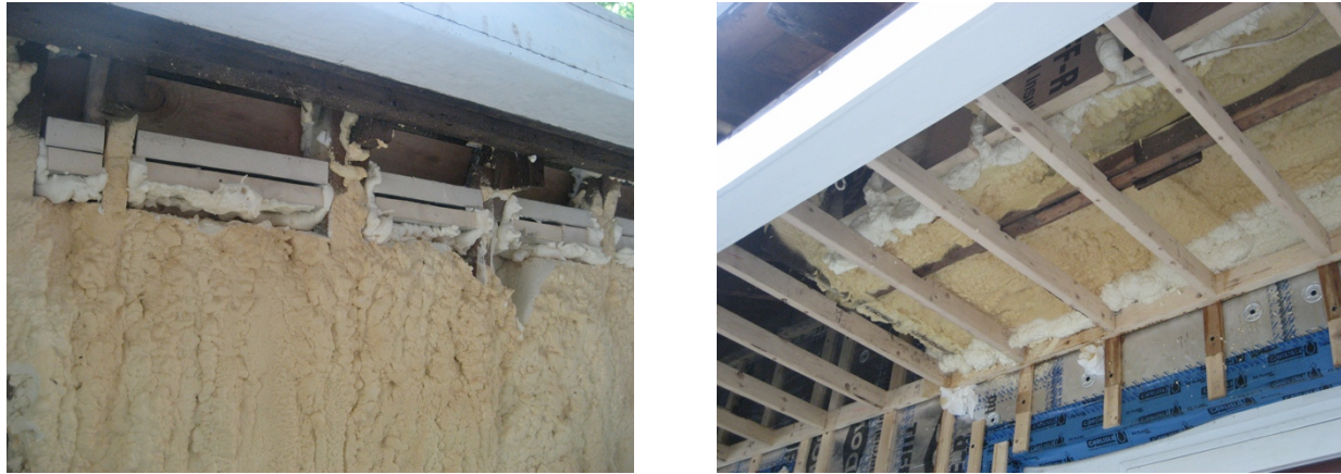
Figure 10. Left: Initial two-part ccSPF application to connect wall insulation to previous work; Right: subsequent two-part ccSPF providing more robust connection.
