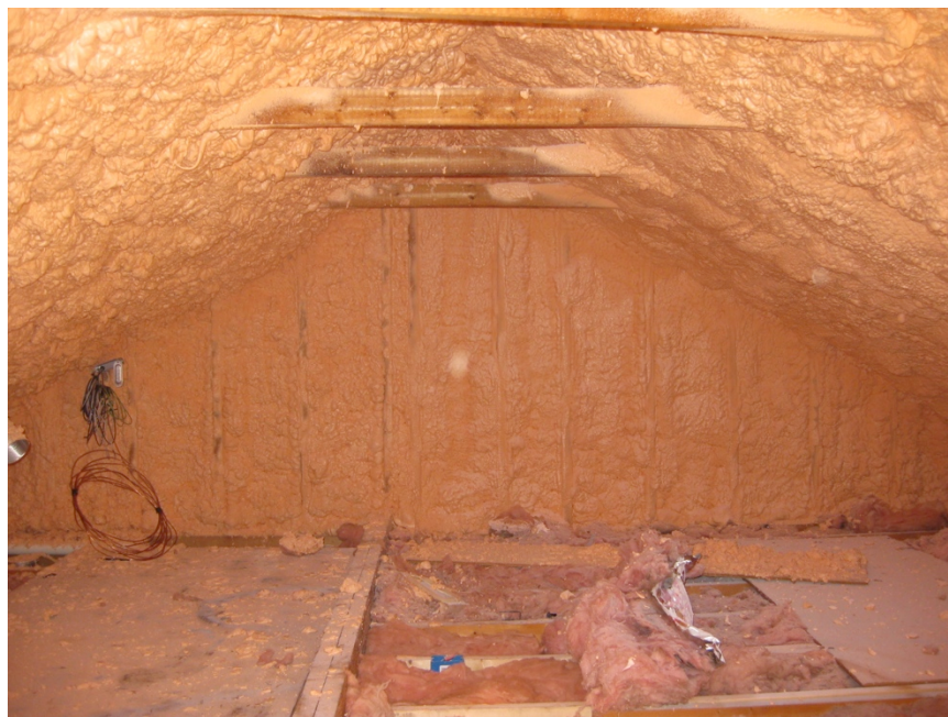
Figure 6. Test home 1 retrofit roof assembly
