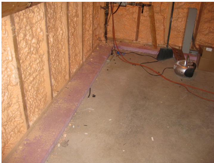
Figure 54. Thermal break between wood stud wall and existing concrete slab at Test Home 1
