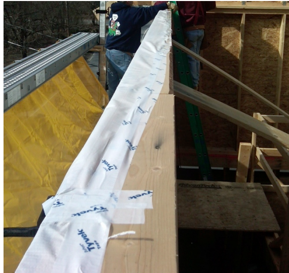
Figure 31. House wrap airflow control transition at top of wall at Test Home 5
