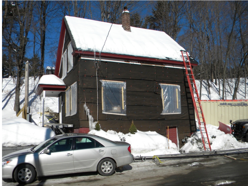
Figure 17. Pre-retrofit Colonial in Lancaster, Massachusetts
