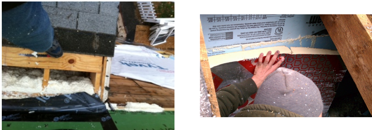
Figure 40. Left: ccSPF airflow control around porch roof framing at Test Home 3; Right: Worker applying rigid foam and foam sealant between attached porch roof and porch ceiling, Test Home 4
