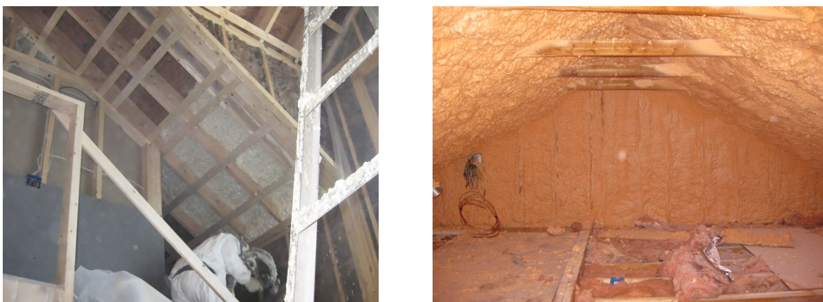
Figure 24. Left: SPF insulation being installed in roof framing cavities at Test Home 3. Note how roof framing precludes insulation for an appreciable portion of the roof area and that the strapping depth does not allow much depth for insulation over the framing; Right: roof rafters fully embedded in spray foam insulation at Test Home 1.
