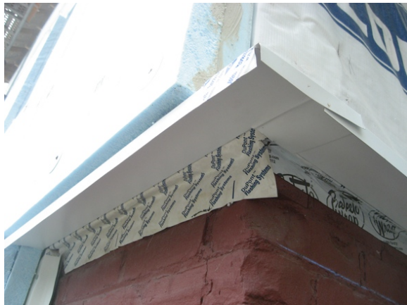
Figure 44. Left: Airflow control transition at existing brick foundation wall, Test Home 5; Right: Airflow control transition at new CMU foundation wall section, Test Home 5
