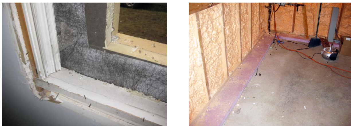
Figure 7. Left: Window opening at Test Home 1 with existing window still in place. Note exterior insulation and house wrap airflow control layers installed to exterior; Right: Basement slab perimeter insulation at Test Home 1.
