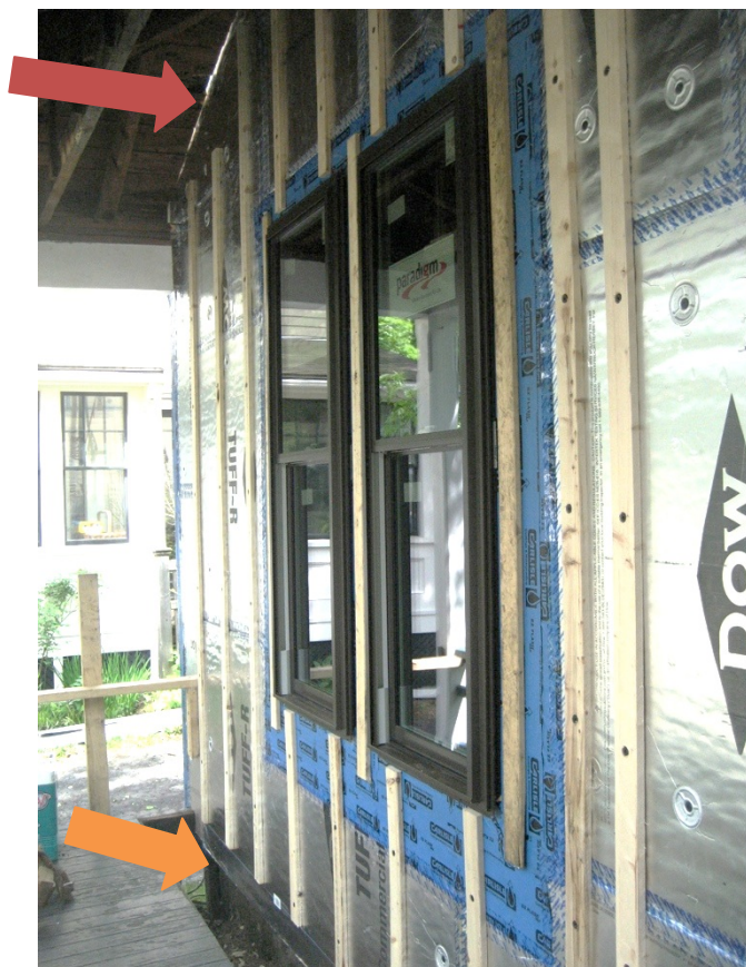
Figure 41. Porch deck, ceiling, and roof cut away from wall to allow continuous air, thermal, and water control, Test Home 2
