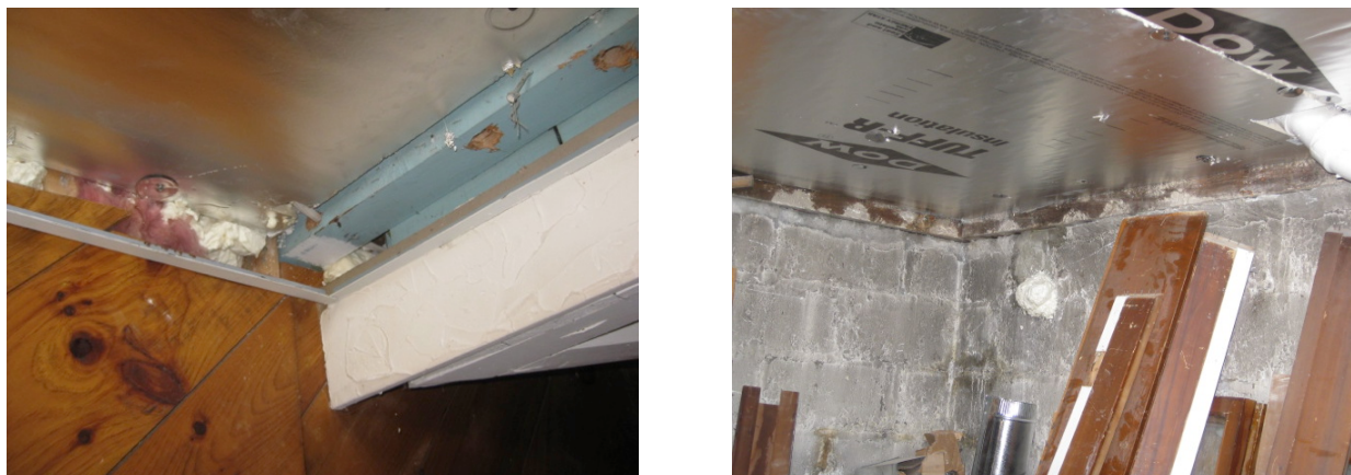
Figure 55. Left: Structural beam exposed to basement; Right: Framed wall sill exposed to basement
