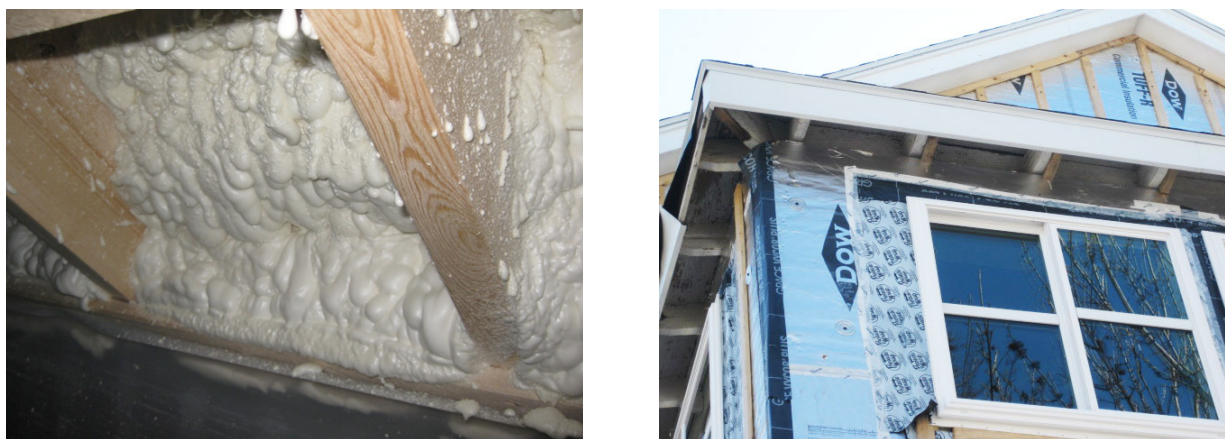
Figure 14. Left: ccSPF providing transition of airflow control at new roof to new wall transition; Right: Rigid exterior insulation notched around projecting rafters.
