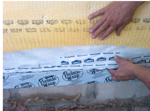
Figure 44. Left: Airflow control transition at existing brick foundation wall, Test Home 5; Right: Airflow control transition at new CMU foundation wall section, Test Home 5
