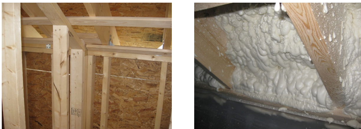
Figure 22. Left: Rafter bay continuous to soffit area at Test Home 3; Right: SPF insulation in rafter bay connecting to top of wall at Test Home 3
