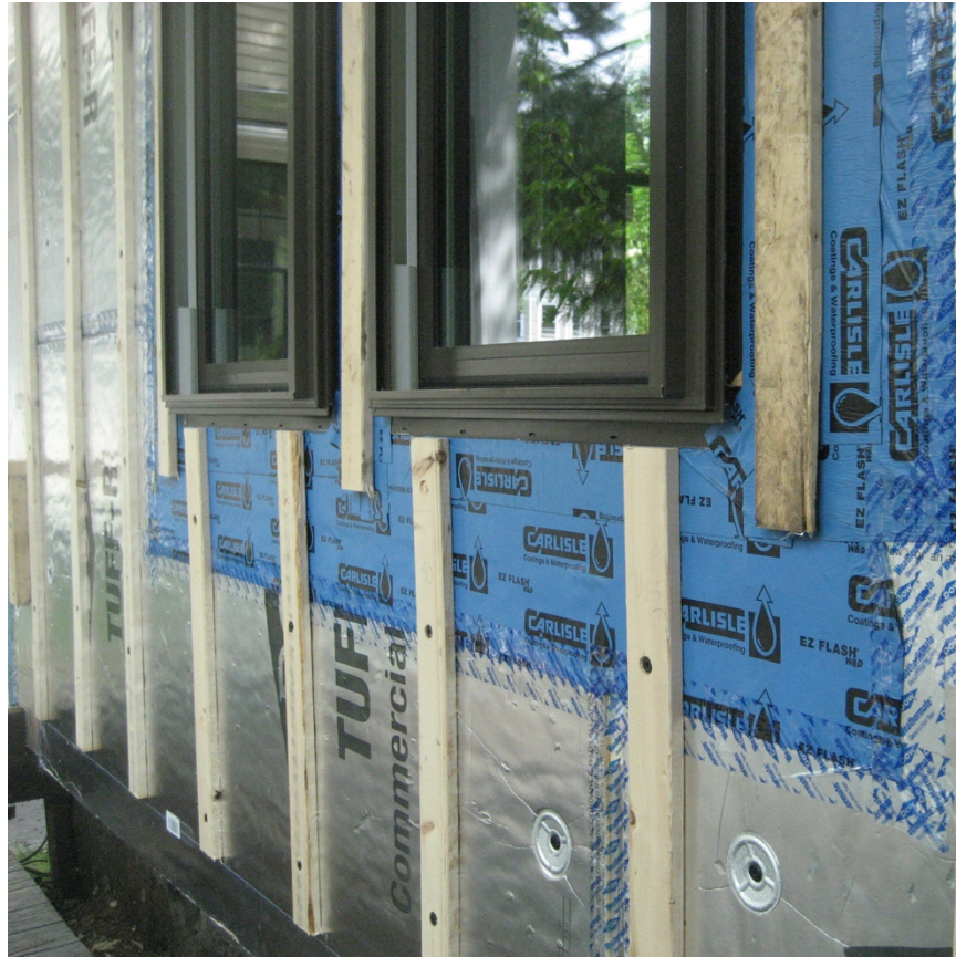
Figure 51. Window installed with flanges aligned with drainage plane at Test Home 2. Note strapping run up to, but not over, bottom flange of window. A single piece of strapping at the side of the window is sufficient to support both trim and cladding attachment.
