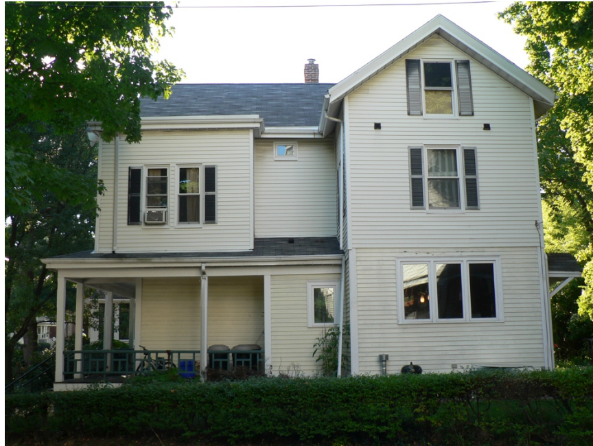
Figure 8. Pre-retrofit Victorian located in Brookline, Massachusetts
