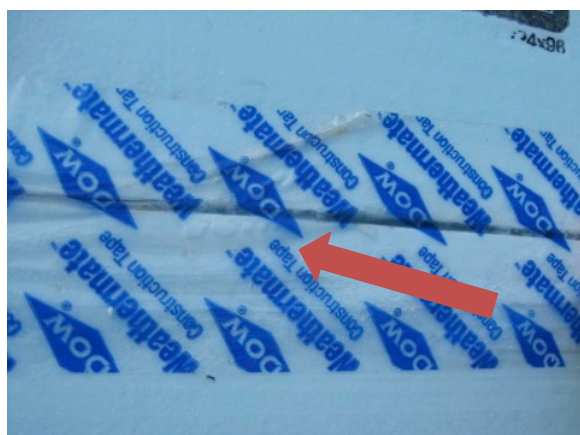
Figure 37. Left: Sheathing tape with water accumulated beneath wrinkle. Right: Fastener for insulating sheathing disrupting water control.
