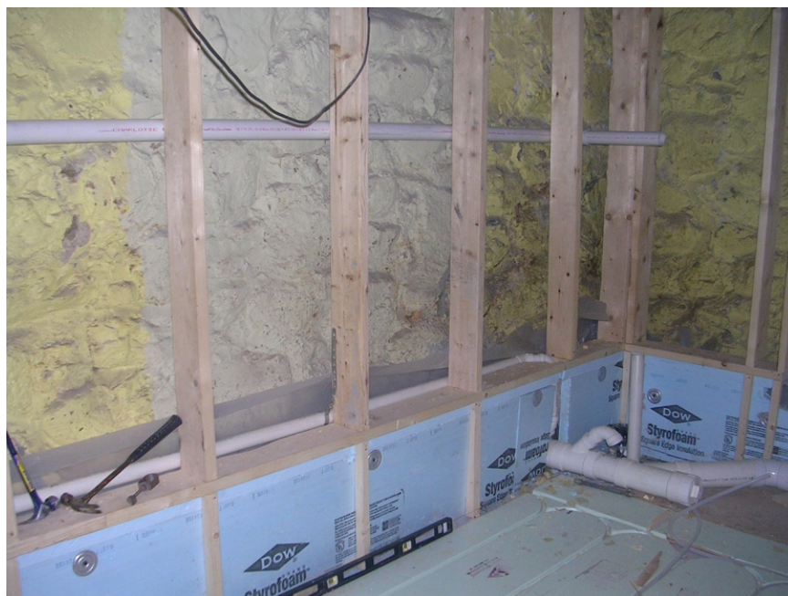
Figure 53. Thermal break between wood stud wall and concrete underpinning wall at Test Home 4
