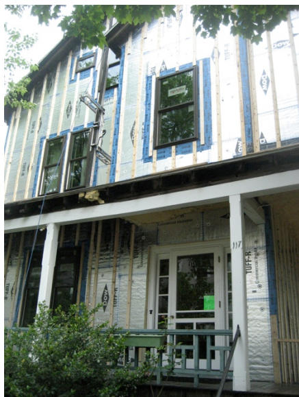
Figure 46. Left: Front of building showing overhang during retrofit work, Test Home 2; Right: connection between new work and previous work at wall-overhang interface, Test Home 2
