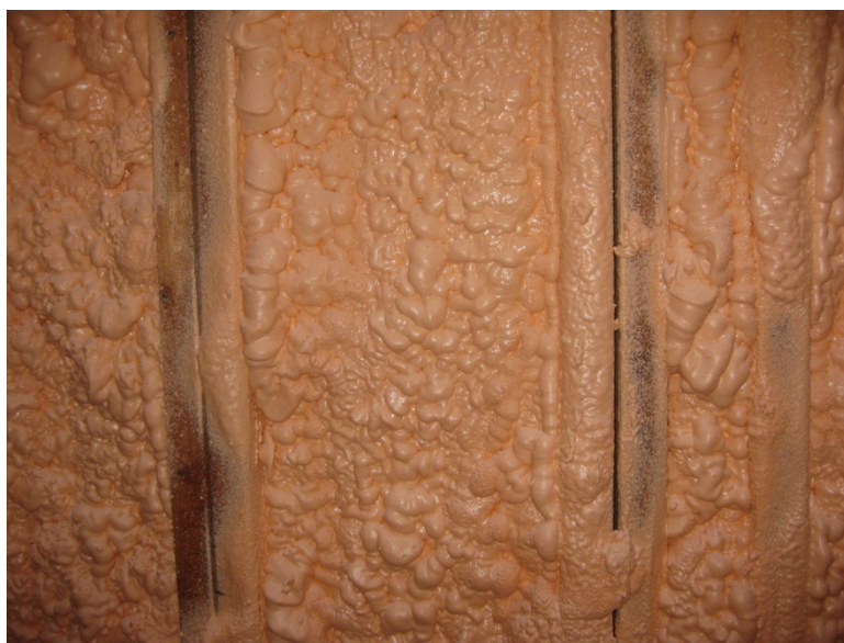
Figure 21. Airflow channels between double roof rafters at Test Home 1
