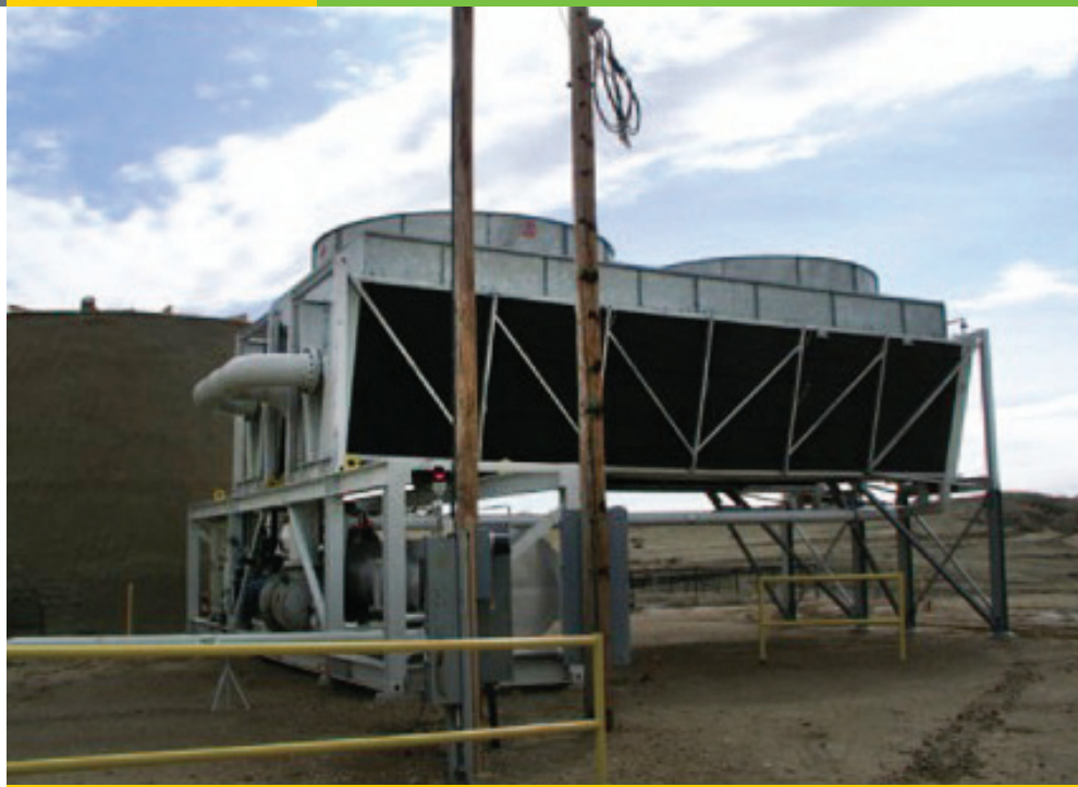
The Rocky Mountain Oilfield Testing Center in Wyoming was one of the first projects to validate the use of co-produced geothermal fluids from oil and gas wells for power generation. The binary cycle plant, shown here, produces approximately 200 kW of electricity.
