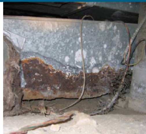
The Building America Pasadena Ranch House case study demonstrates the value of beginning with an energy audit. Illustrated here is an open plenum discovered in the crawlspace ( www1.eere.energy.gov/buildings/building_america/hot_dry_mixed_case_studies.html ).
