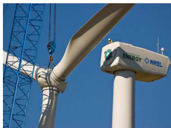
Figure 10. Installation of DOE 1.5 MW turbine
