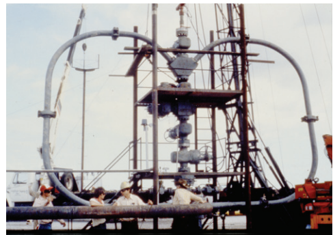
Figure 28b. To accommodate the high brine flow rate, a block “Y” was installed on the production wellhead.
