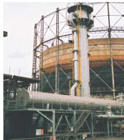
Figure 19 – Kalina Cycle - Installation -
