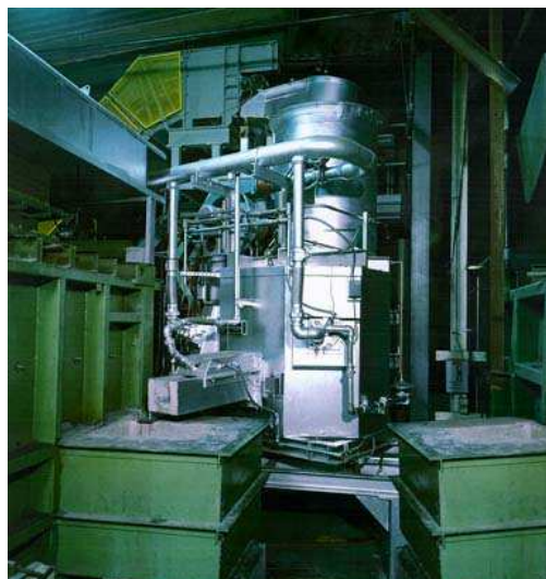
Figure 12 - Stack Melter in a Die - Casting Facility -
