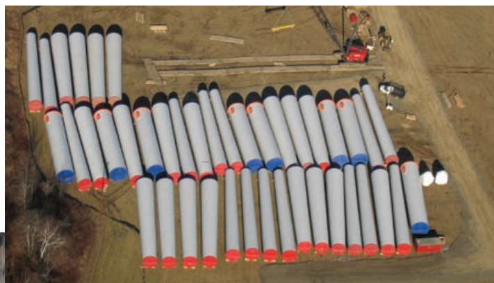
Blades and towers for the Stetson Ridge Wind Project await installation. (Photo credit: Dave Wilby, IEPM/PIX15571 at left, and PIX15572 above)
