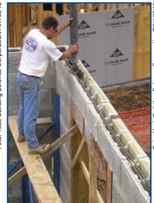
The wood fiber-cement block was selected for its ability to handle moisture in the building enclosure.
