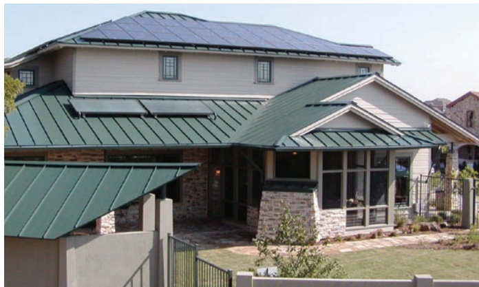
Great unobstructed southern exposure for the photovoltaic and solar water panels, the “engines” of this Zero Energy Home.
