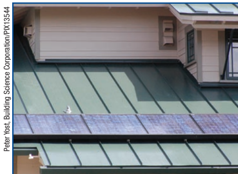
Outside air intakes are neatly tucked under a second story eave.
