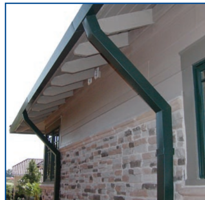
Durability is all in the details—wrap-around overhangs, recessed windows, fibercement siding and trim, gutters, bath exhaust vents.
