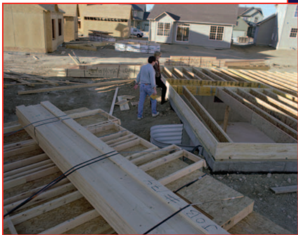
Prefabricated wall panels await assembly at the Meadow View community in Longmont, Colorado. McStain Enterprises is the builder partner (IBACOS).
