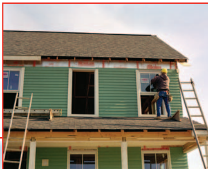
Warren Gretz, NREL/PIX04670
