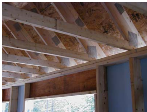
Figure 1-7. A "slider" truss
