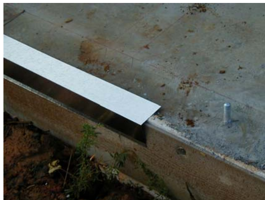
Figure 4-5. Flashing with FiberCement board
