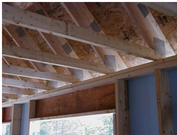
Figure 2-16. A “slider” truss
