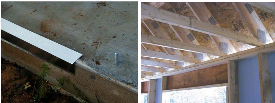
Figure 3-13. Flashing (left) and slider trusses (right)
