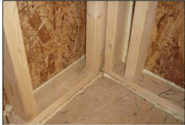
Figure 39. Low-expansion foam used to air seal stud cavities
