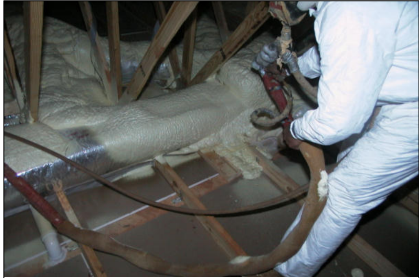
Figure 52. Insulating ducts with closed-cell polyurethane foam
