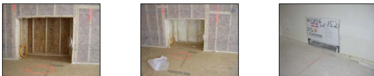
Figure 45. Fireplace bump outs are frequently missed when insulation is installed
