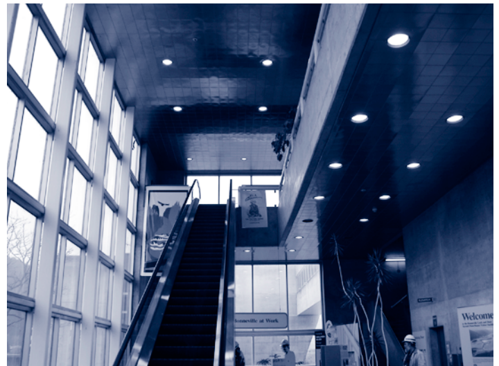
Mercury vapor lighting was replaced with induction lighting in Bonneville Dam's Visitor Center Complex lobby.
