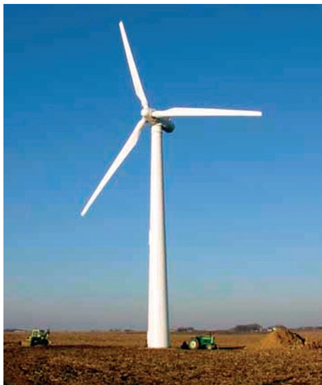
The Bonus 450-kW turbine, newly installed and in operation on a cloudless day in January 2005.
