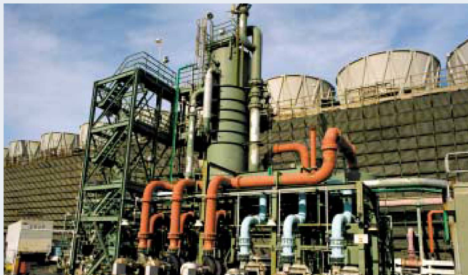
Condensers and cooling towers rise above a power plant at The Geysers.
