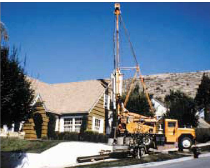
A well is drilled at a residence in Klamath Falls, Oregon, for geothermal direct-use heating.
