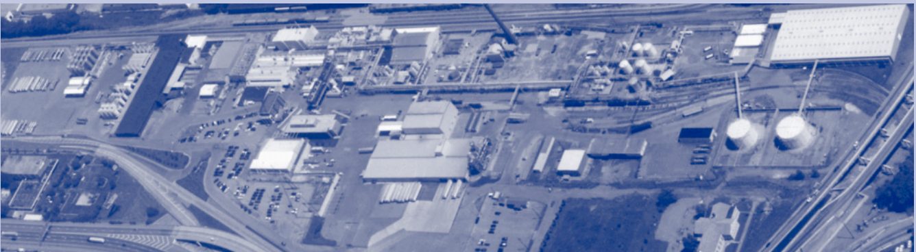
Rohm and Haas' Knoxville Plant
