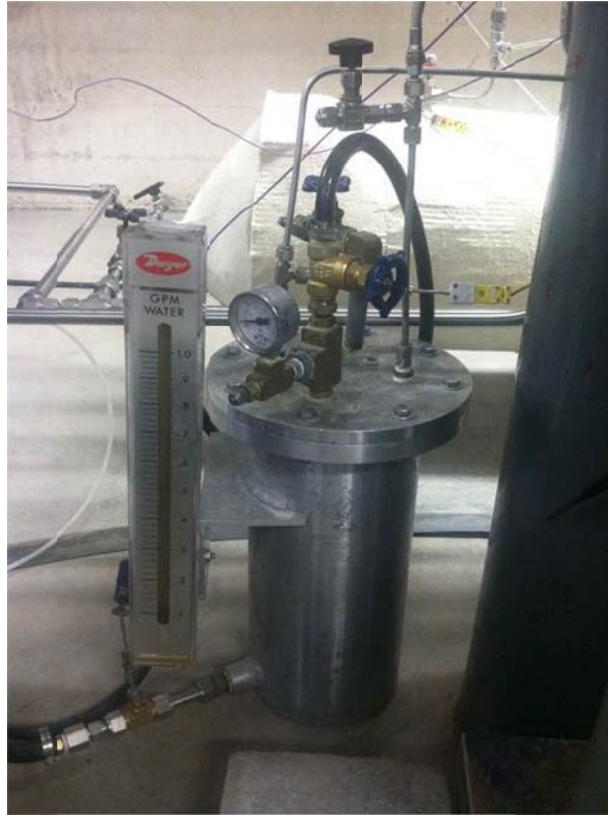
Figure 11. Precooler heat exchanger utilizing chilled water.
