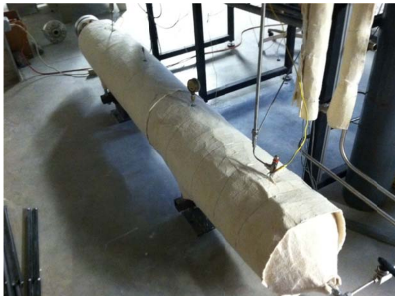
Figure 10. Heated and insulated buffer tank used to reduce pressure fluctuations from compressor shifting.
