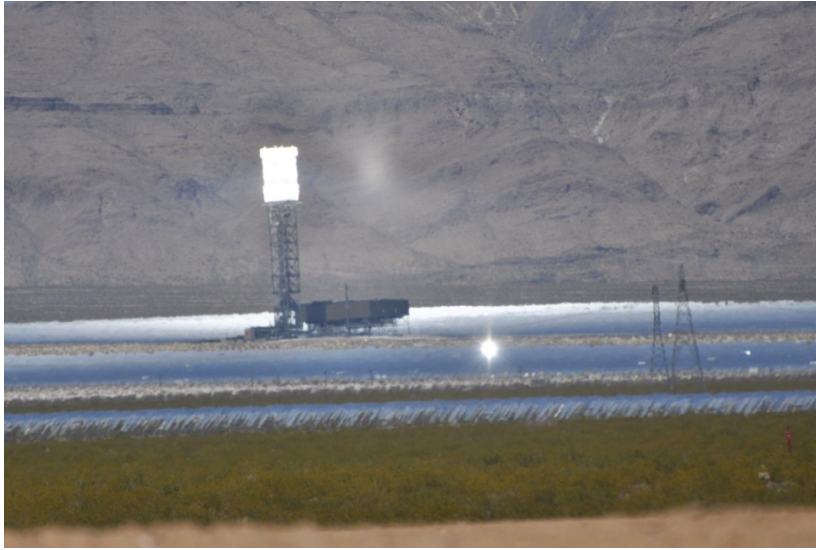
Fig. 8. Photograph of Unit 3 receiver and “rogue” heliostat from I-15 (~3 miles away).
