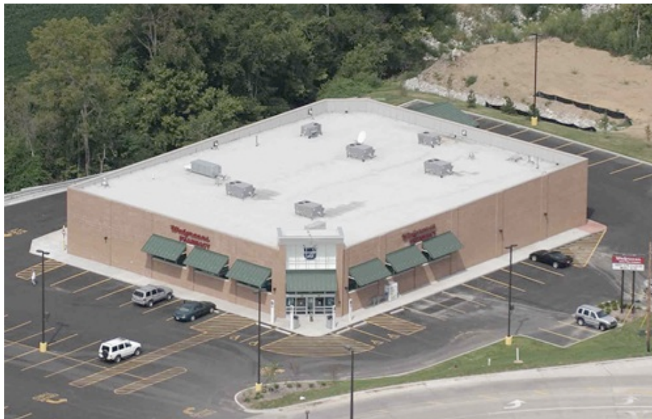
Figure 1: A typical medium-sized building with roof top unit (RTU) heating, ventilation, and air conditioning systems.
