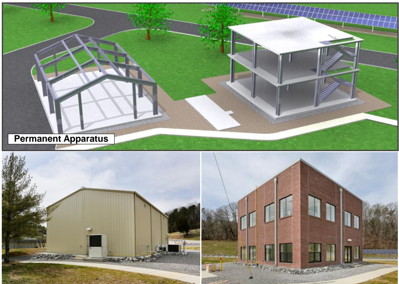
Figure 1 FRP permanent apparatus (above), single-story test FRP (lower left) and 2 story test FRP (lower right)
