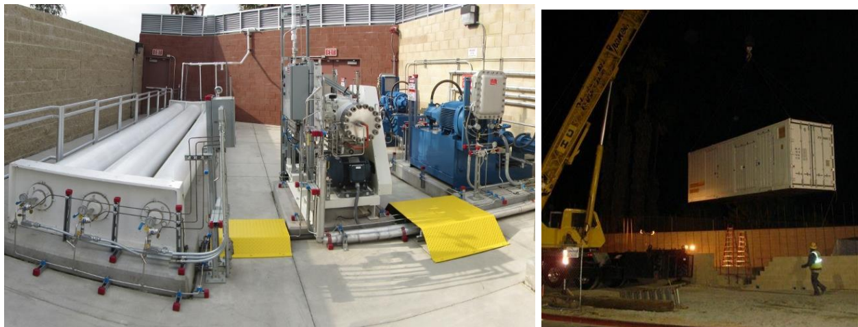
Figure 2. CSULA Hydrogen Station equipment procured with this funding. Left: storage tanks and three compressors. Right: electrolyzer is being installed.
