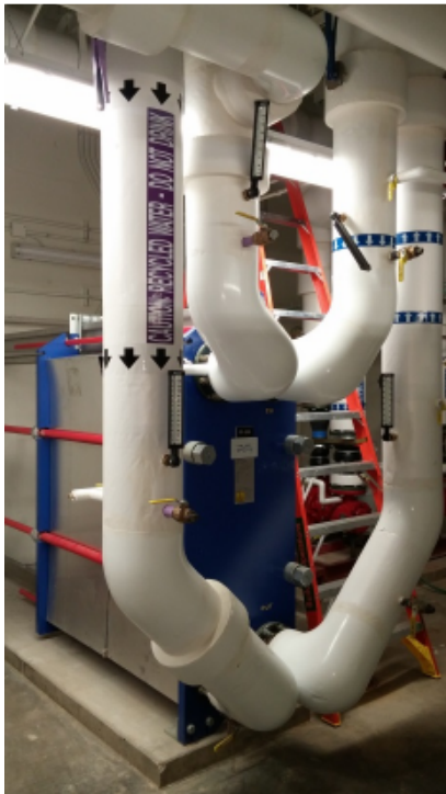
Figure 14: Recycled Water Heat Exchanger
