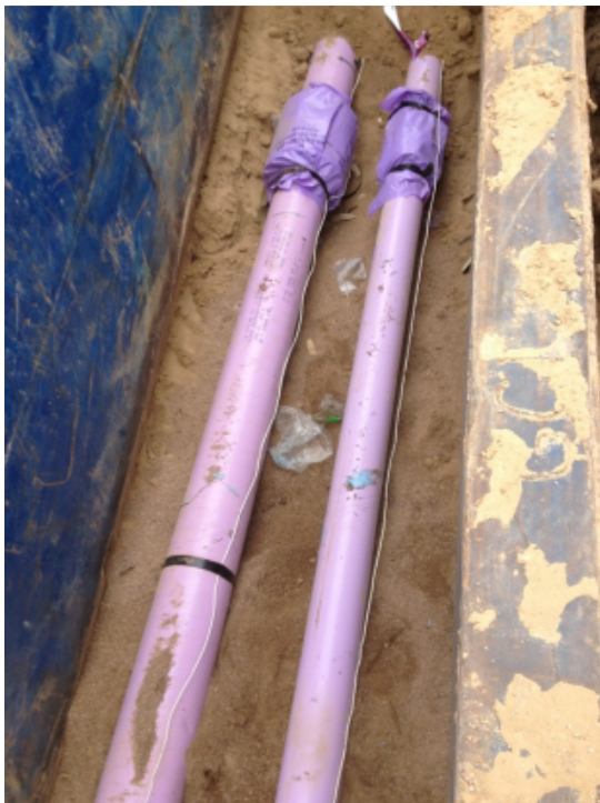
Figure 10: Recycled Piping - Supply and Return Lines
