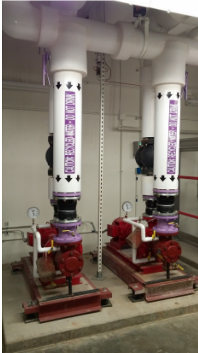
Figure 13: Recycled Water Pumps
