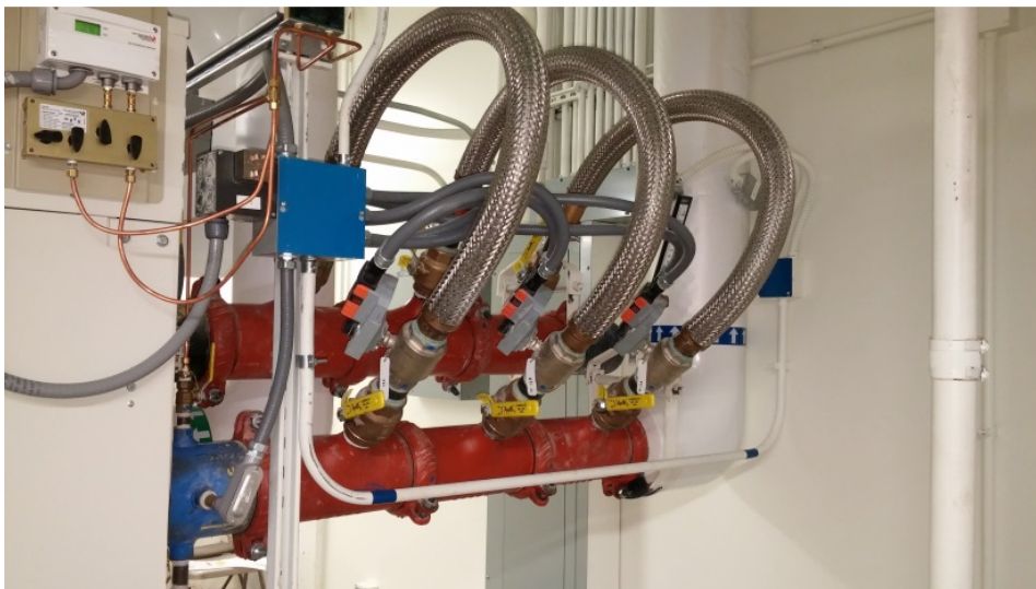
Figure 12: Heat pump Header Bypasses
