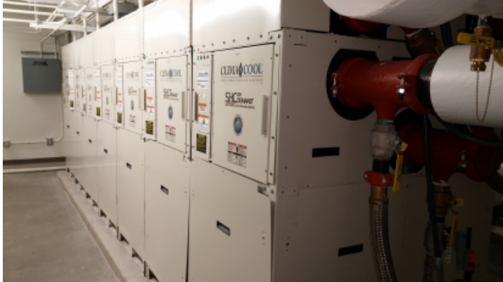
Figure 11: Climacool heat pumps (7 units)
