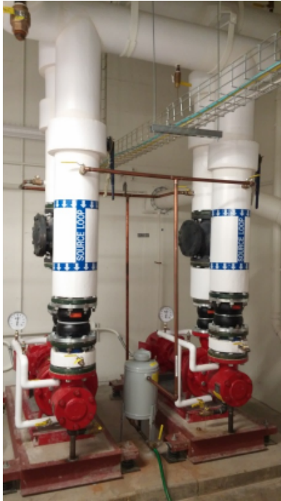
Figure 15: Source Loop Pumps
