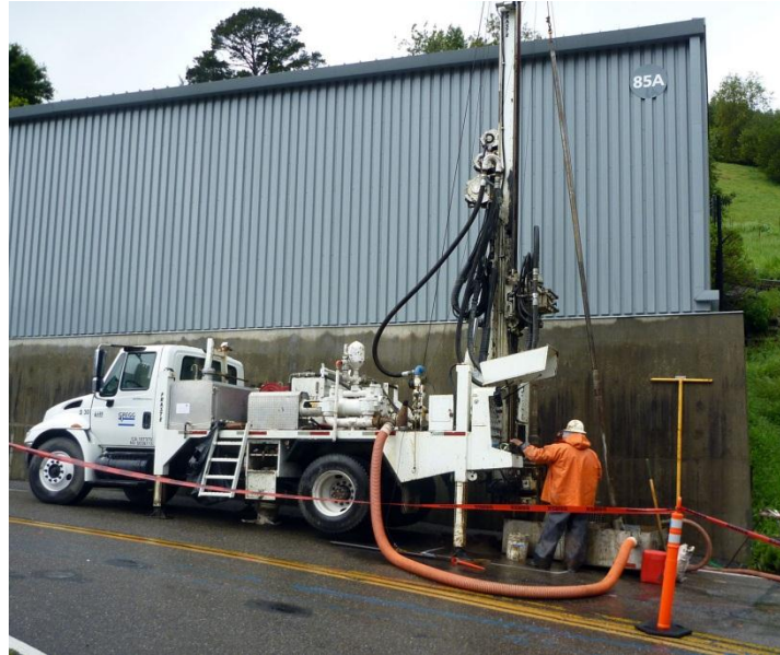
Figure 4-5. Drilling of WF3 along the edge of Calvin Road and Building 85A
