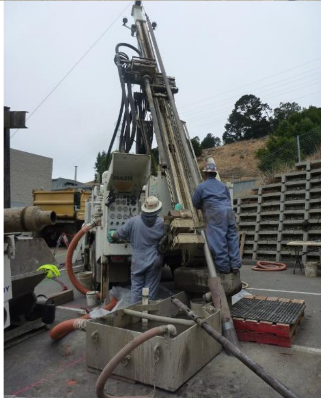
Figure 3-16. Drilling of WF-4. Note that it is a 60° inclined drilling.
