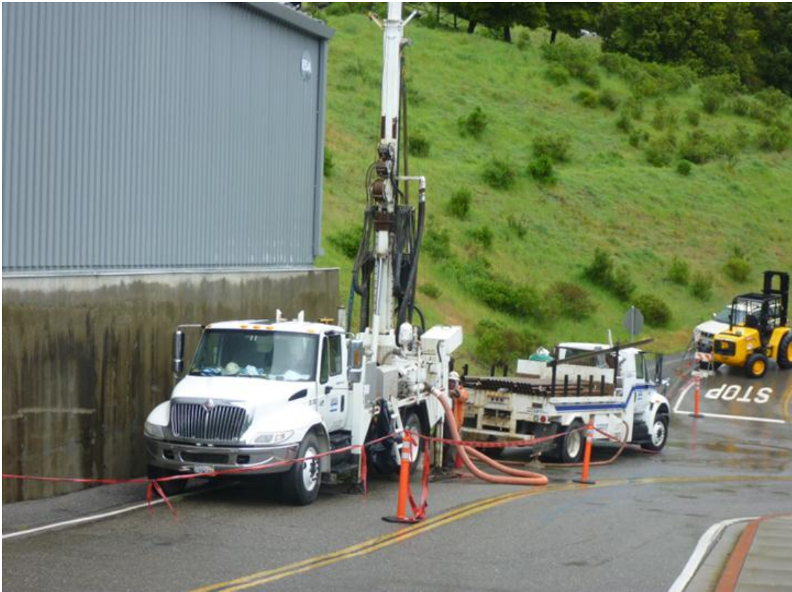
Figure 3-3. Drilling of WF-3. A truck mounted drill-rig with a 30ft mast is used. The truck behind it is the support water truck with drill pipes.
