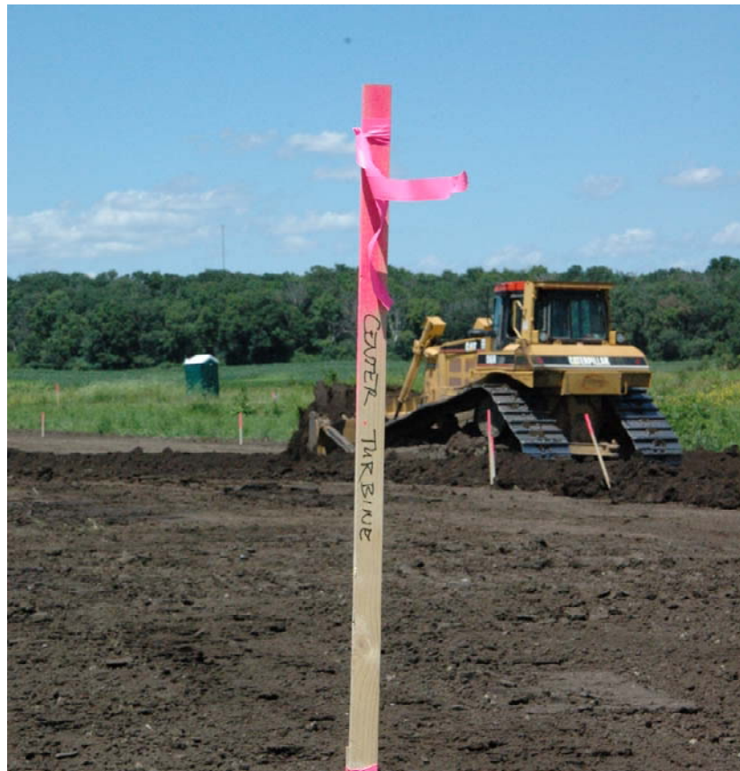
Figure 1.1: Photo of the survey stake marking the location of the wind turbine on the first day of construction. A bulldozer is shown grading the site in preparation for excavation for the foundation.
