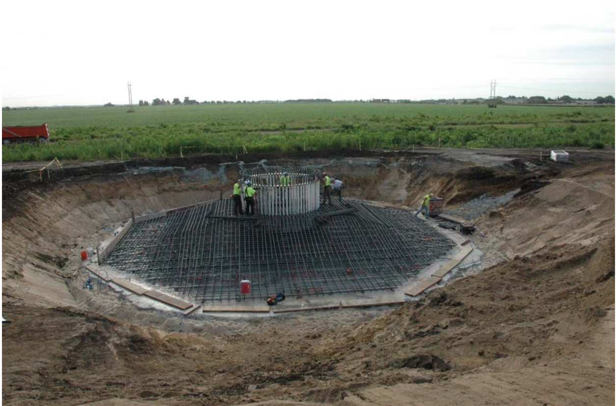
Figure 1.2: The rebar cage of the wind turbine foundation nears completion in July, 2011.
