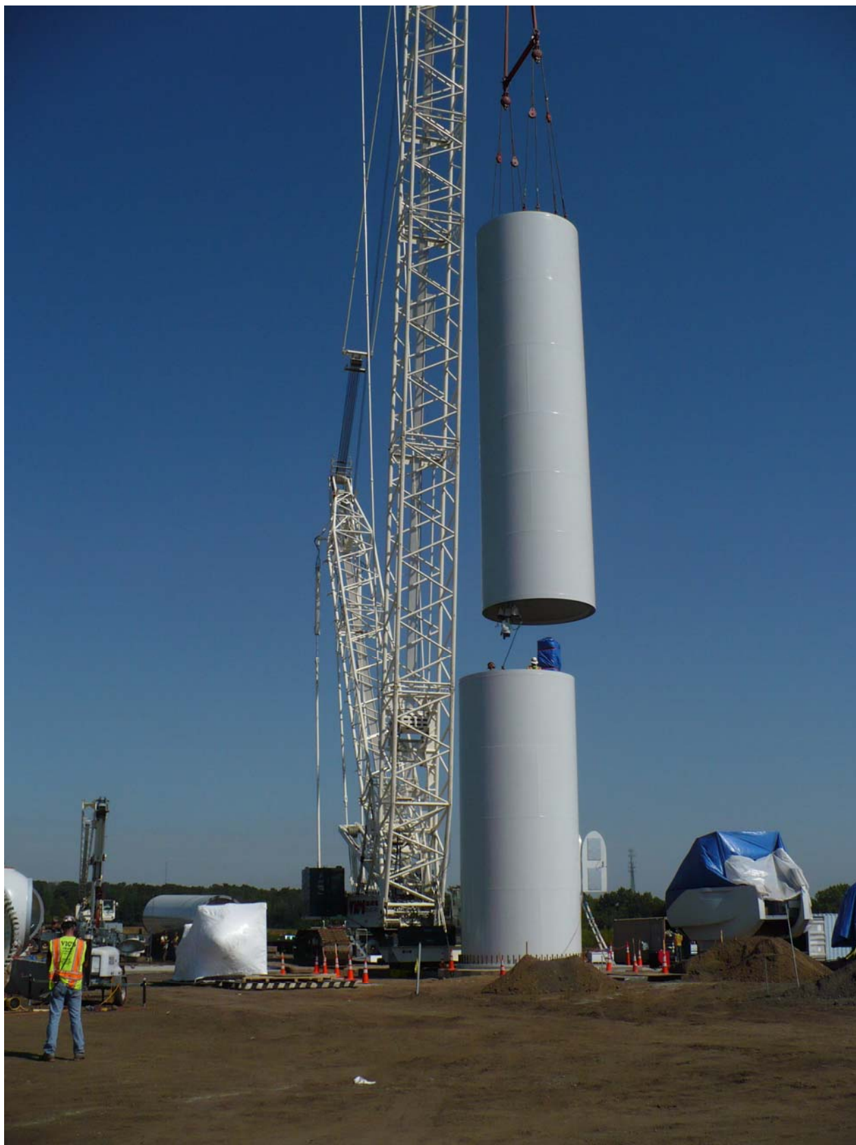
Figure 1.5: The second of four wind turbine tower sections is lifted into place.
