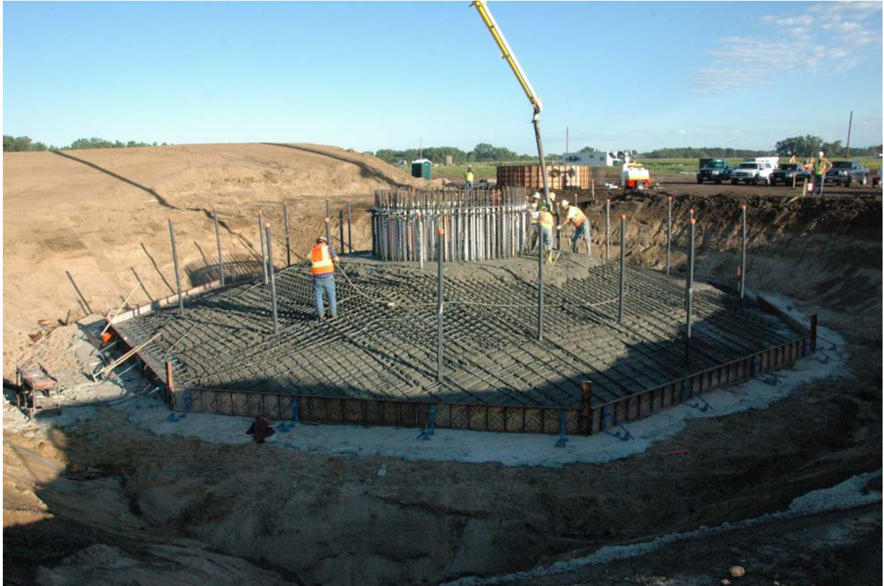
Figure 1.3: Concrete is poured for the foundation of the wind turbine.
