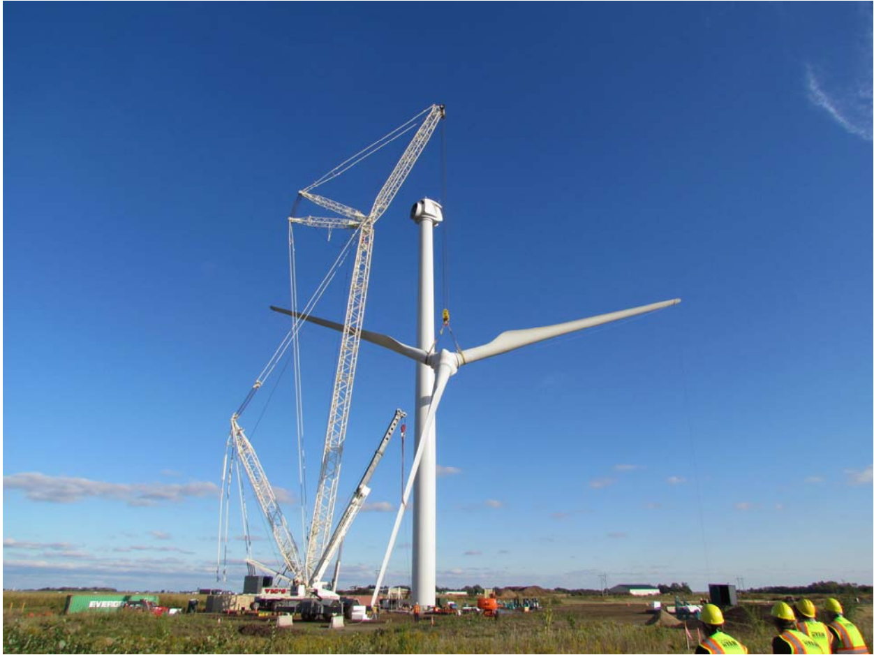
Figure 1.6: The wind turbine rotor is lifted into place on September 23, 2011.
