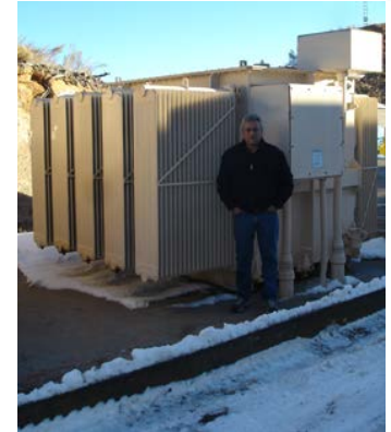
Refurbished Transformer Rectifiers
