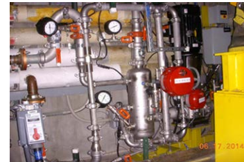
New DTL pumps and control valves
