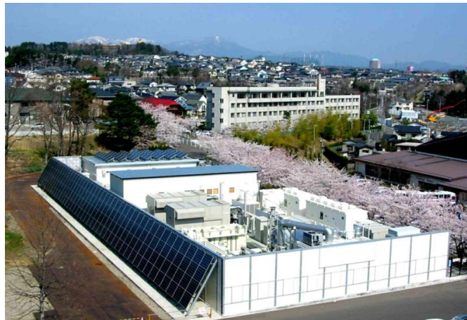
Figure 4: Overhead view of the Sendai energy center
