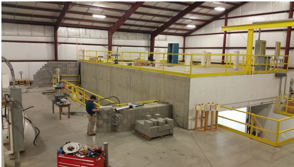
Figure 3. The high-power test facility at the Niowave headquarters. The two tunnel layout with roof access for cryogenics served as the model for the isotope production facility at the Lansing, Michigan airport.
