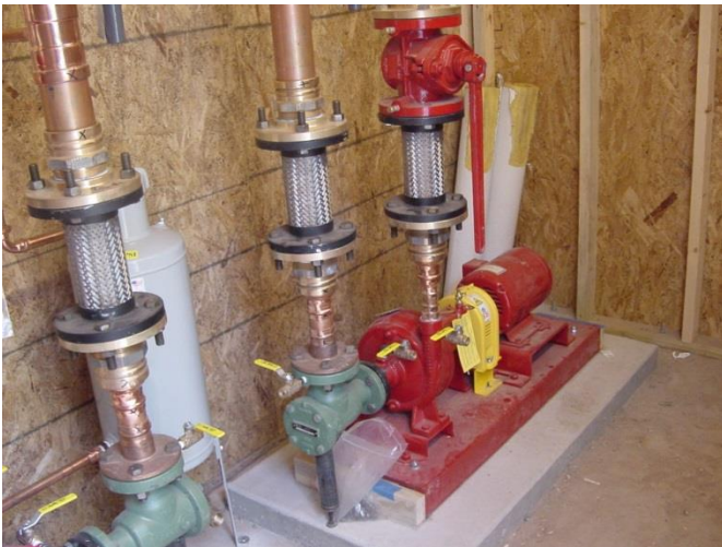
Figure 9 – Pump for Geothermal System
