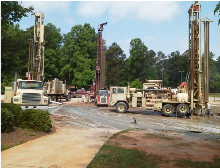
Figure 3 – Drill rigs installing vertical wells in North Village parking lot
