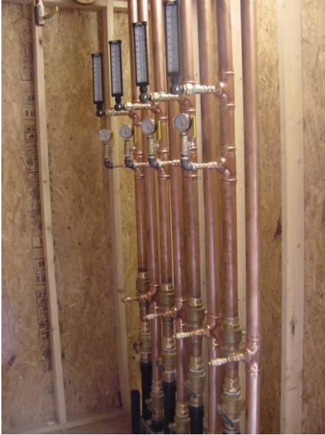
Figure 8 – Piping Manifold
