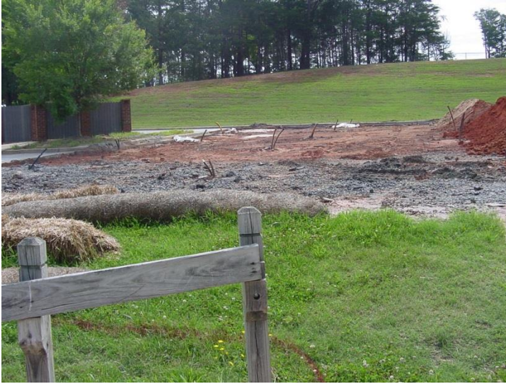
Figure 5 – Well field that shows the plastic tubing protruding from vertical well.
