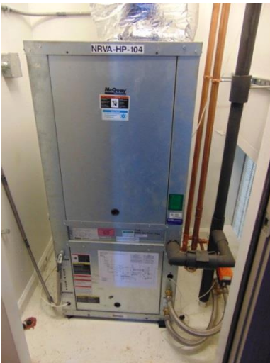
Figure 11 – 2.5 Ton Geothermal Heat Pump
