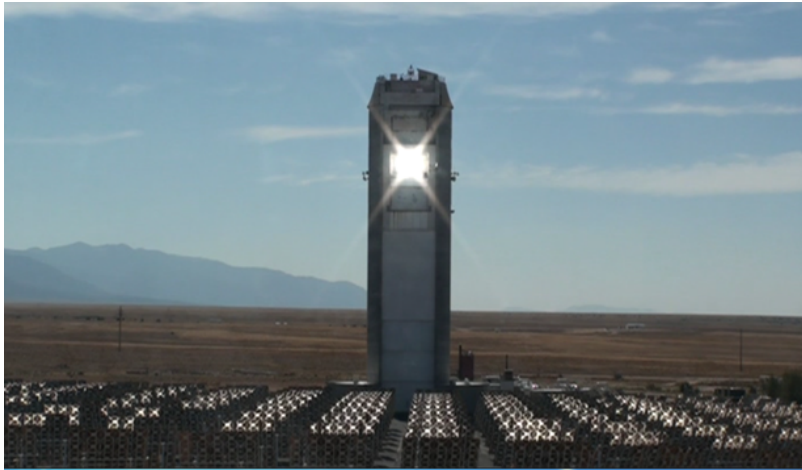
(a) Solar energy concentrated on the test bay used for these tests
