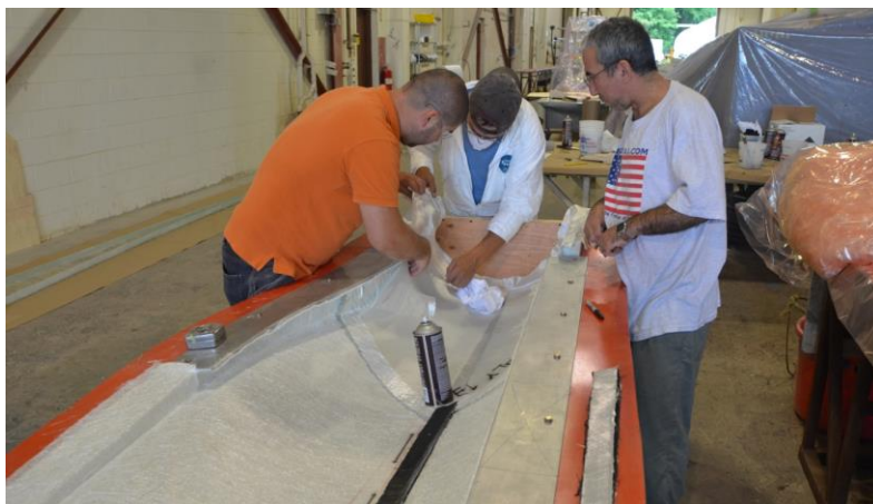
Figure 6: Workers at TPI laying up dry, fiberglass fabric for a BRC test blade.
