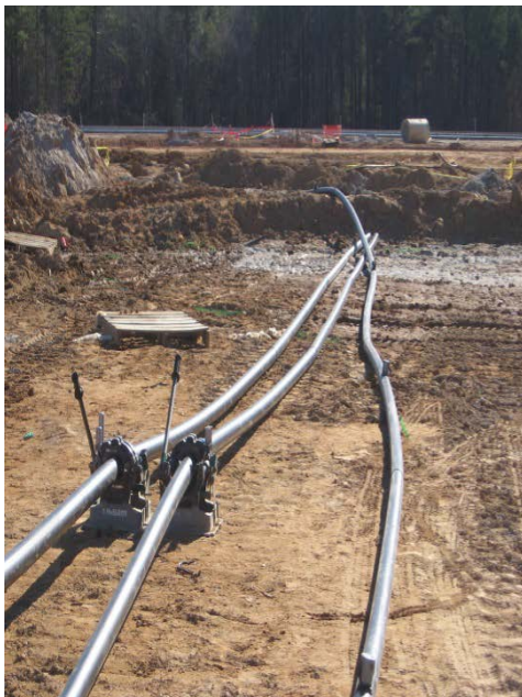
Header Pipe Thermal Welding
