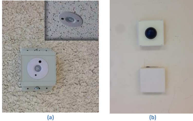
Figure 32 (a) Photosensors; (b) temperatures (top: operative, bottom: air)
