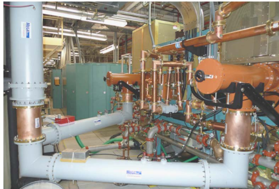
Figure 2: Coaxial feeders from PAs to branch hybrid
