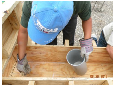
Fig. 5.34 Apply form release oil
