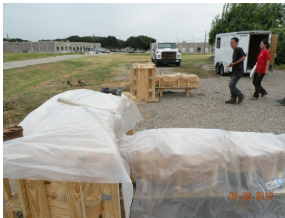
Fig. 5.39 Curing of concrete
