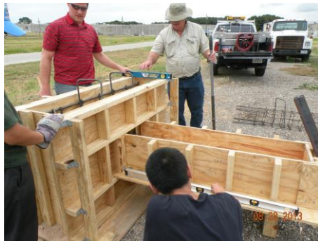
Fig. 5.33 Level formworks
