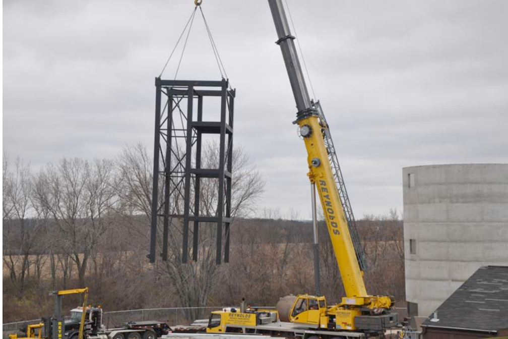
Figure 99 – Support structure being lifted into silo.
