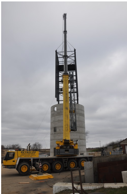
Figure 100 – Support structure lowered into silo.
