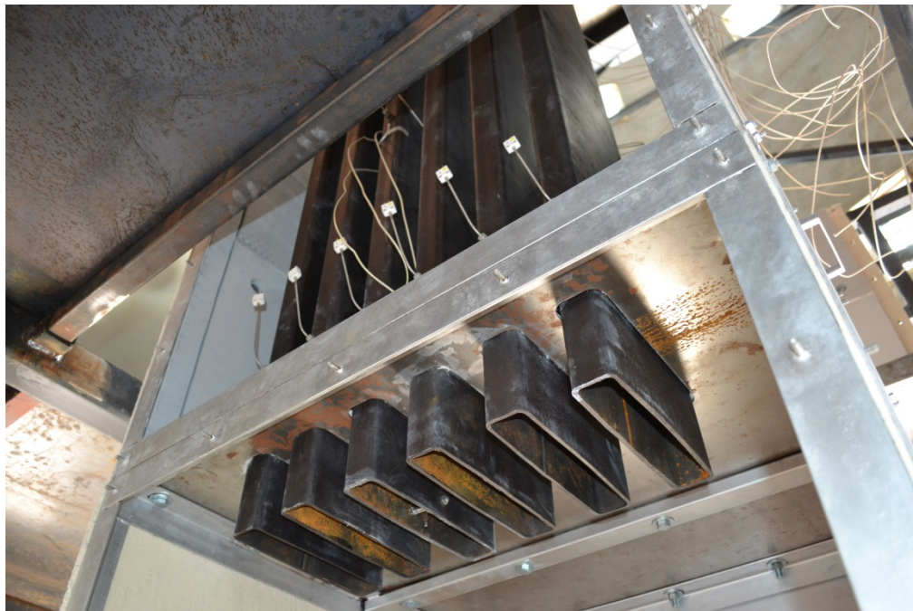
Figure 108 – Painted riser ducts inserted into cavity.
