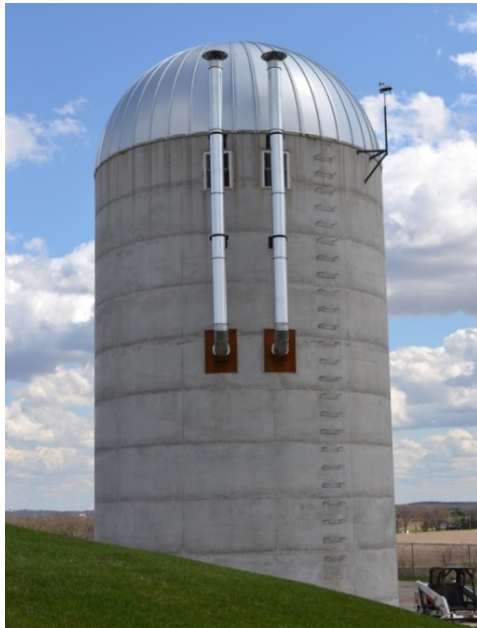
(a) Silo exterior
