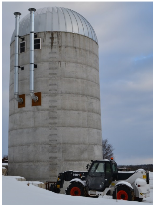
Figure 21 – Exhaust ducts on silo exterior.
