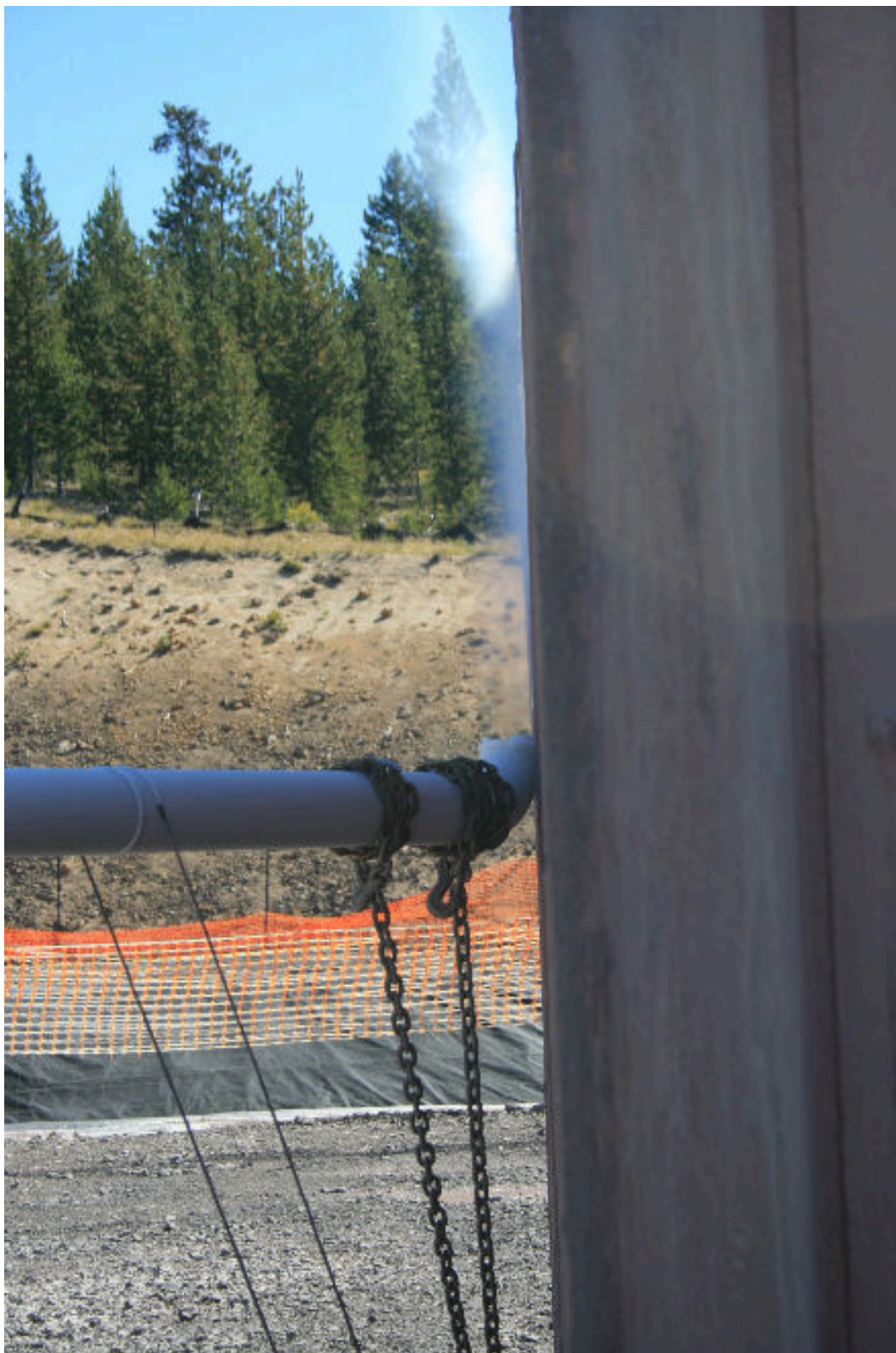
Figure 9: Initial gas flow from well NWG 46-16. Note the endothermic reaction of gas decompressing, resulting in frost forming on the flow line when the valve is first opened (8 September 2013).
